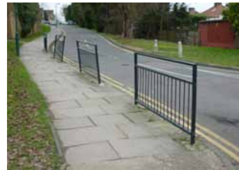
Single panels of guardrail should never be used
