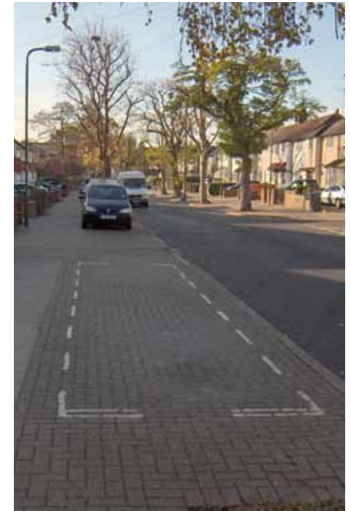
Full footway parking bay
