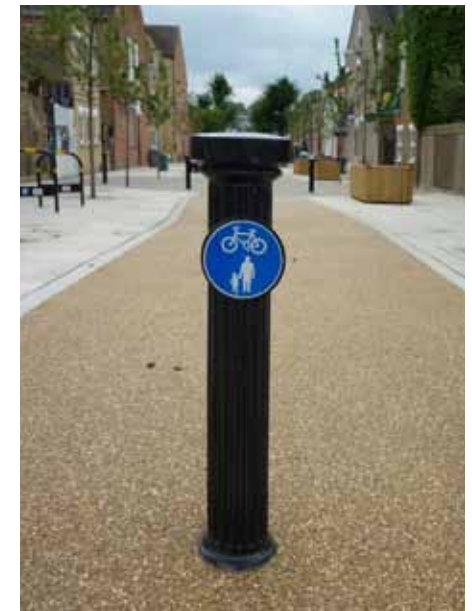
Bollard incorporating signage
