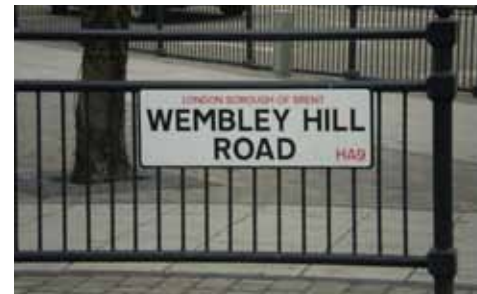
Guardrail incorporating signage
