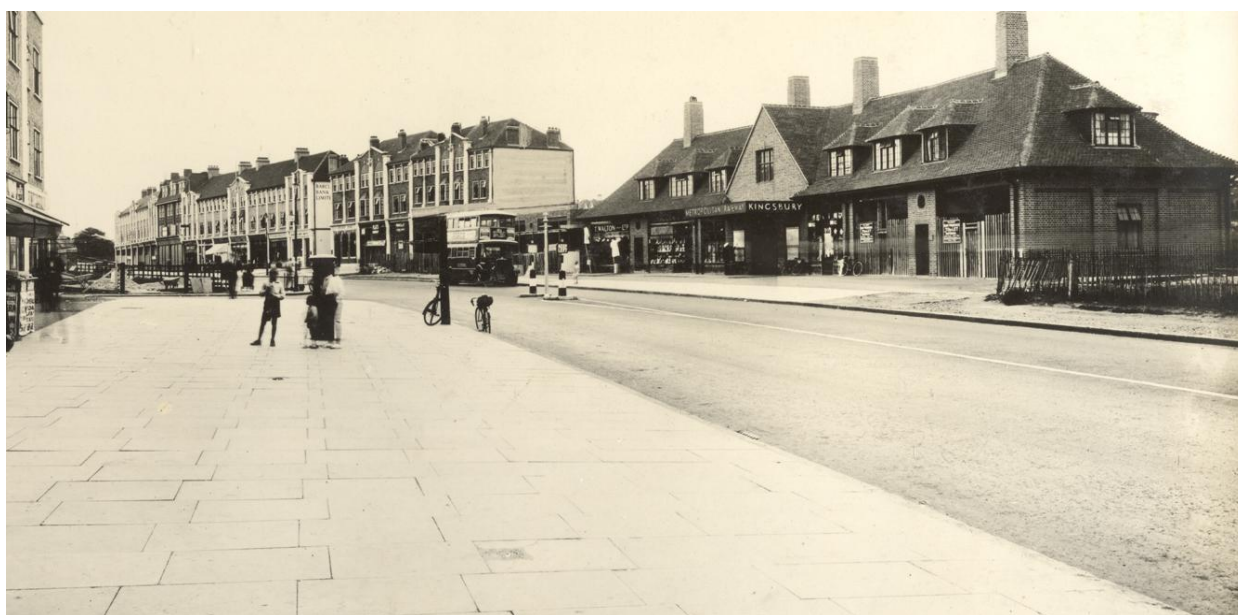
Kingsbury Road, with the new station and a 183 bus, in the summer of 1933.
