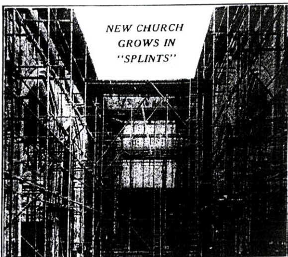
A MAZE OF STEEL scaffolding at present encloses St. Andrew's Church, Kingsbury, the fabric of which has been removed from St. Andrew's, Wells Street, W. It is anticipated that the work will be finished in the early autumn.
