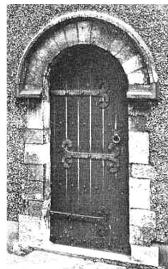
The restored “Saxon” door > [Photo by Philip Grant, 2009]
