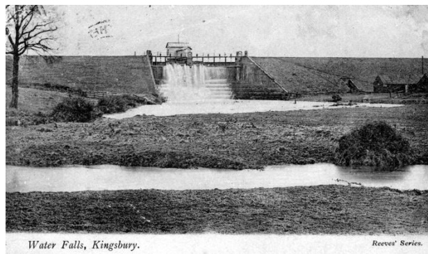
Water Falls, Kingsbury.
