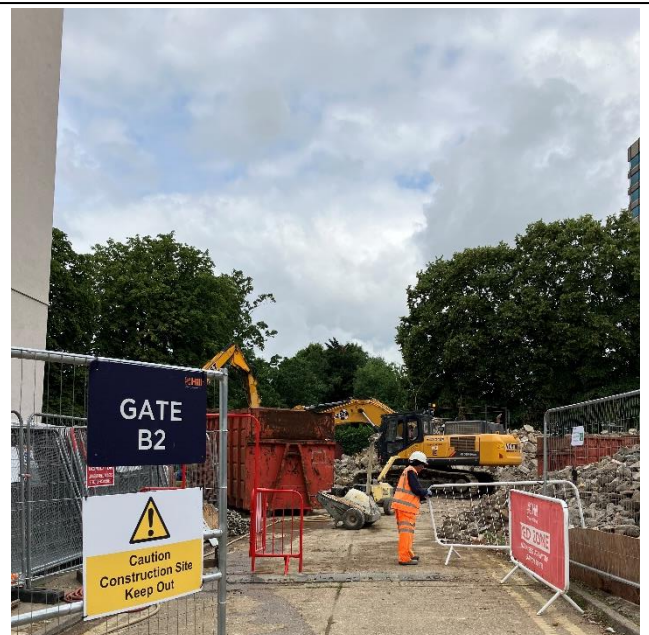
Demolition Of Claire Court
