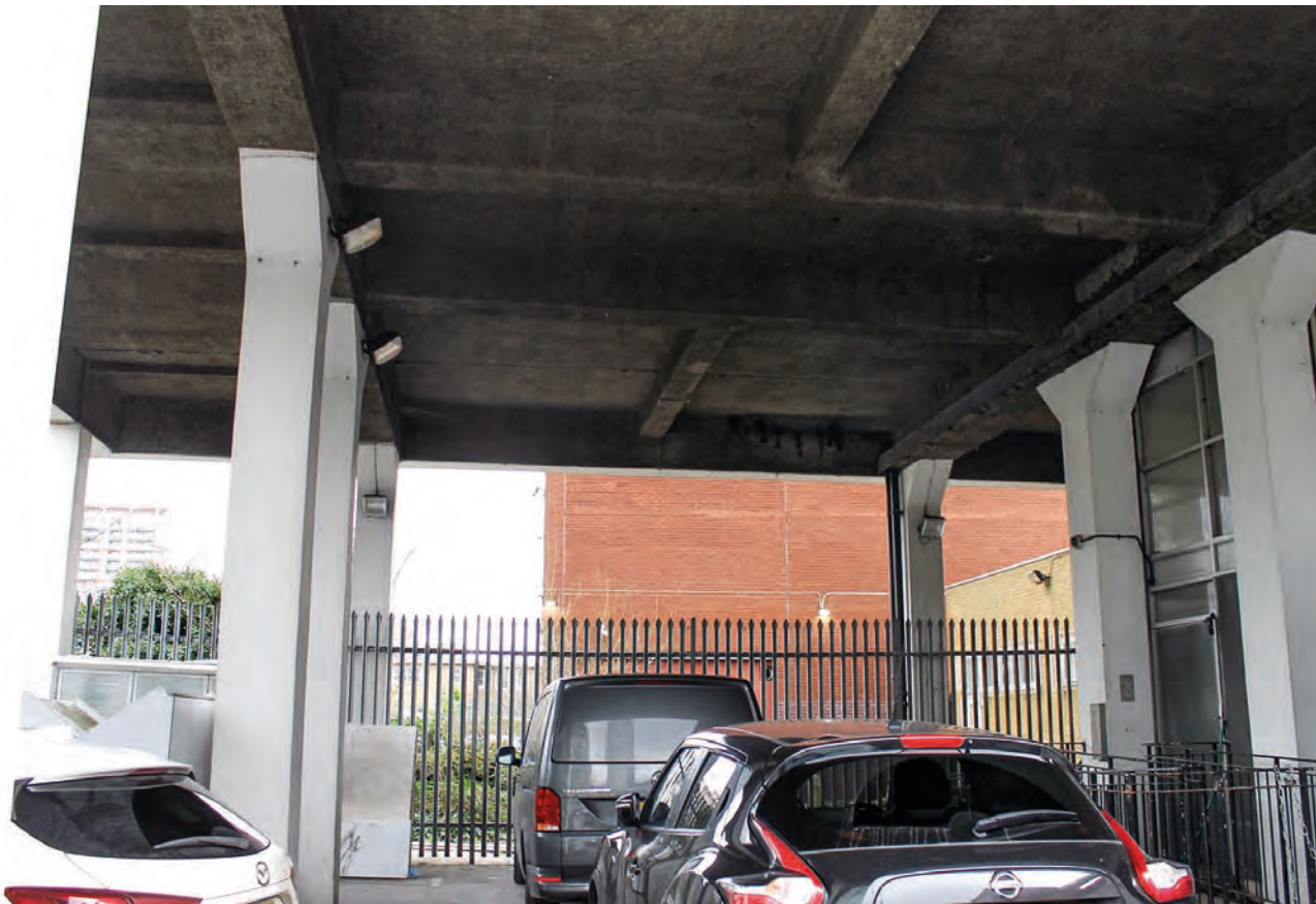
Plate 4: View to rear of Fairgate House, looking east
