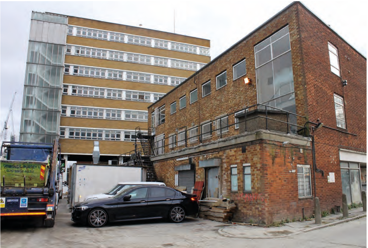
Plate 5: View to rear of Pitman House and Fairgate House, looking east-south-east
