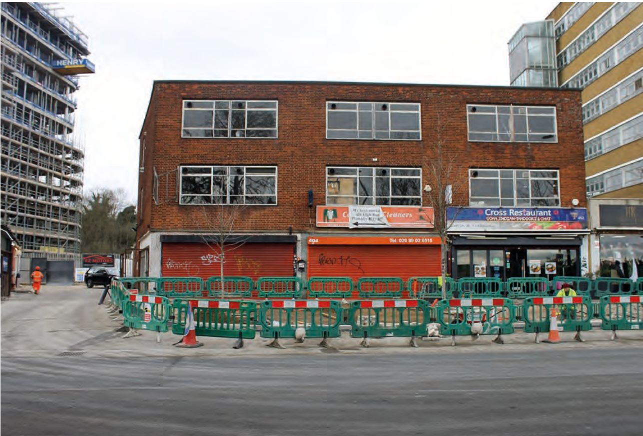
Plate 1: Pitman House and side access road, looking north
