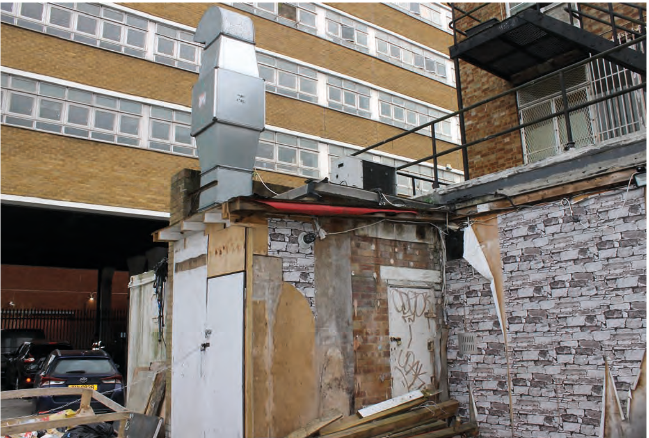
Plate 6: Brick wall and extension to rear of Pitman House, looking south-south-east
