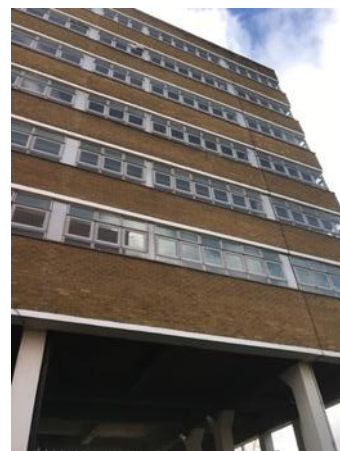
Photo 6: East elevation of seven-storey structure
