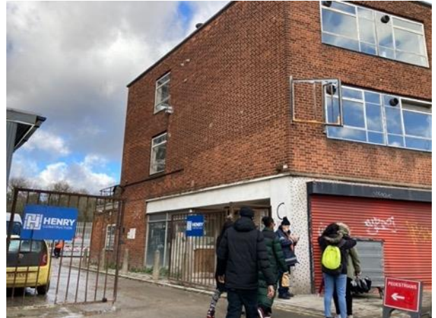
Photo 2: Western elevation of the three-storey buildings
