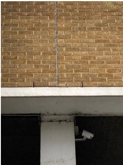
Photo 9: Weep holes within the brickwork
