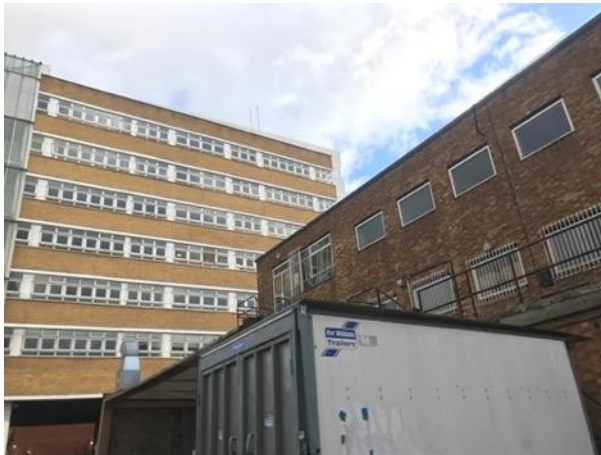
Photo 3: Northern elevation of the three-storey building and western elevation of seven-storey building
