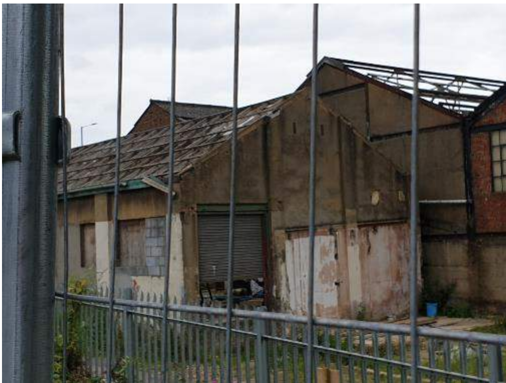
Figure B.18 B3 exterior
