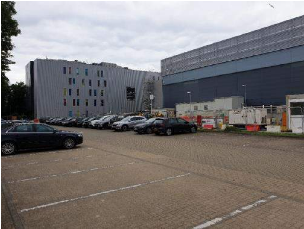
Figure 4.12 Hardstanding on site
