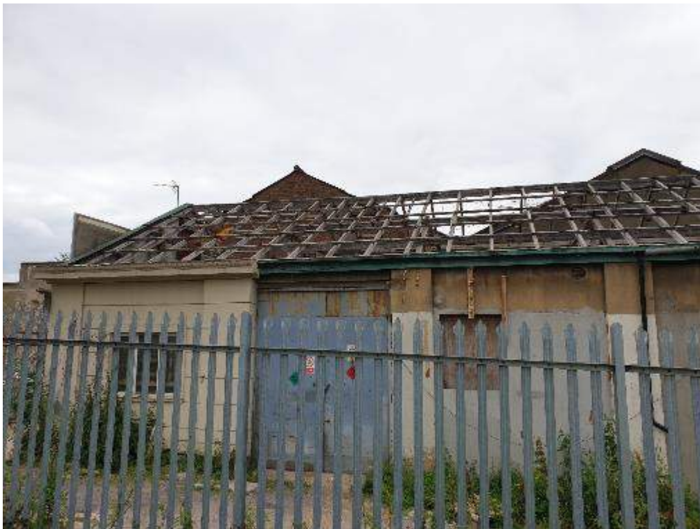
Figure B.17 B3 exterior
