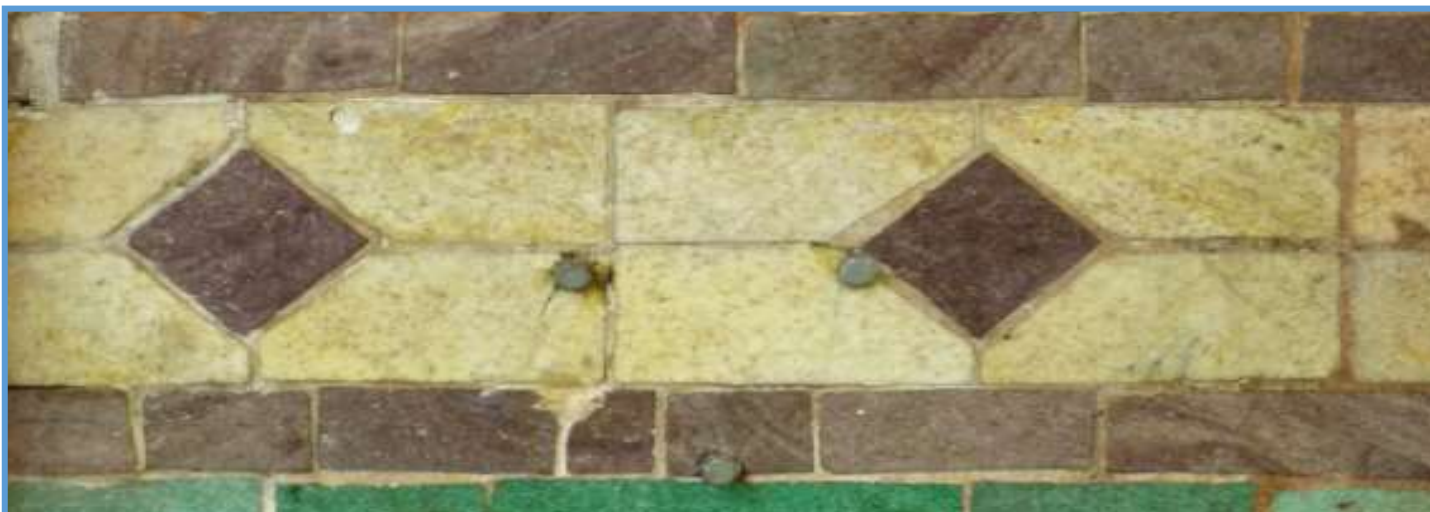
Detail of the glazed bricks within the ticket office at the Grade II listed Willesden Underground station. 1925 by Charles Walter Clark, architect for Metropolitan Railway Company.
