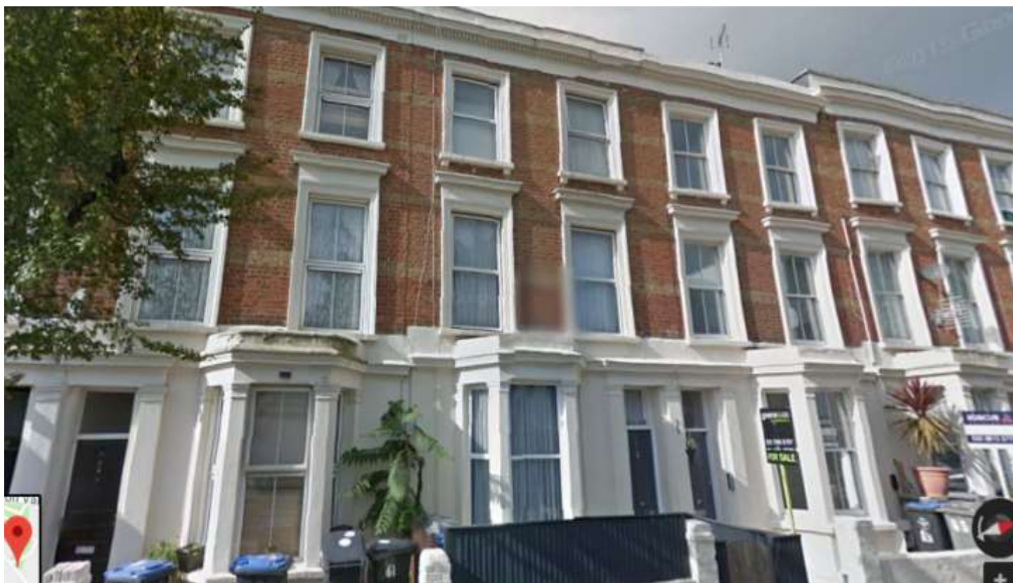
Attractive and well-preserved terrace housing with brick and stucco detailing
