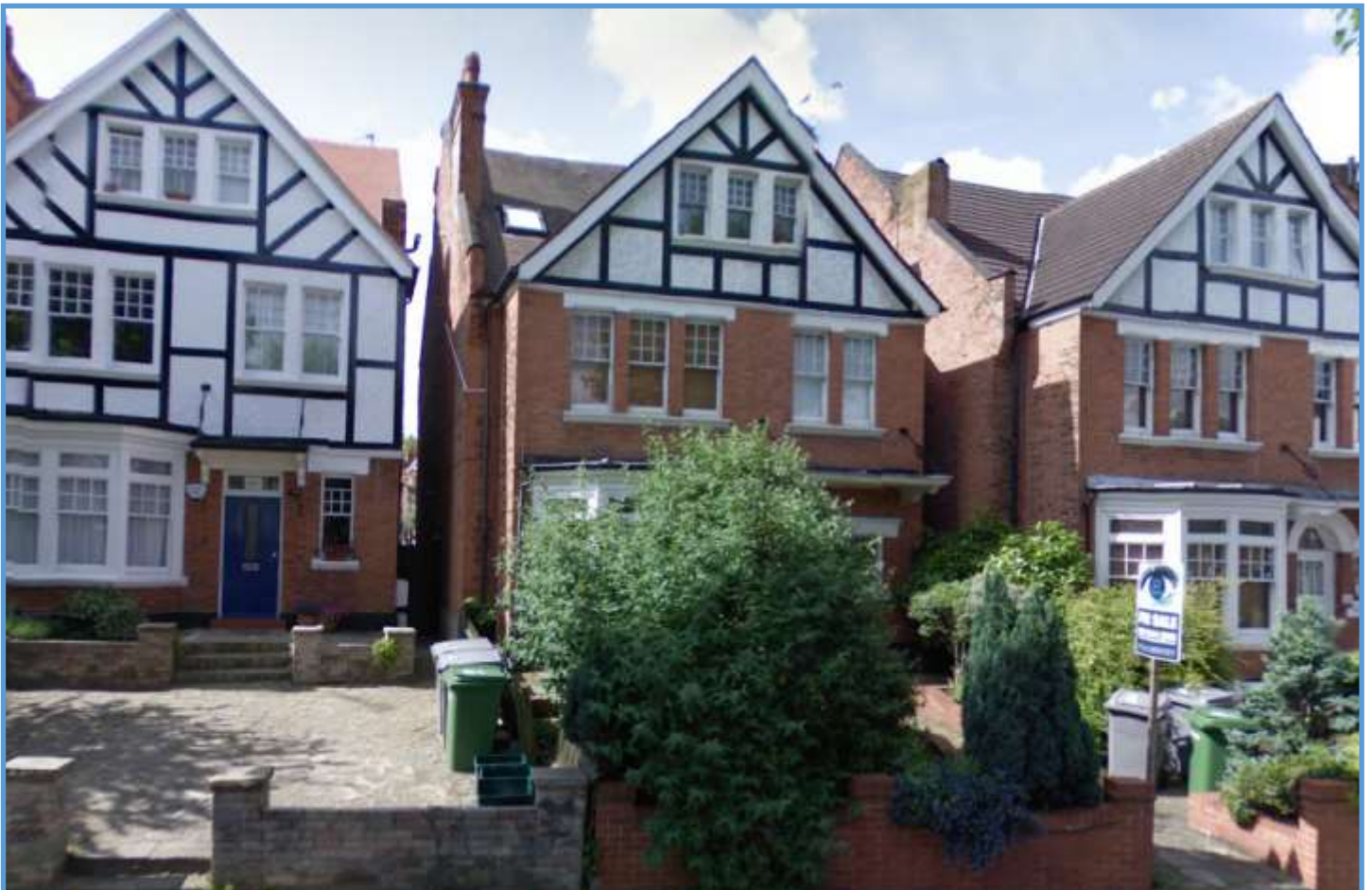
Possible boundary extension to the Willesden Green Conservation Area along Brondesbury Park
