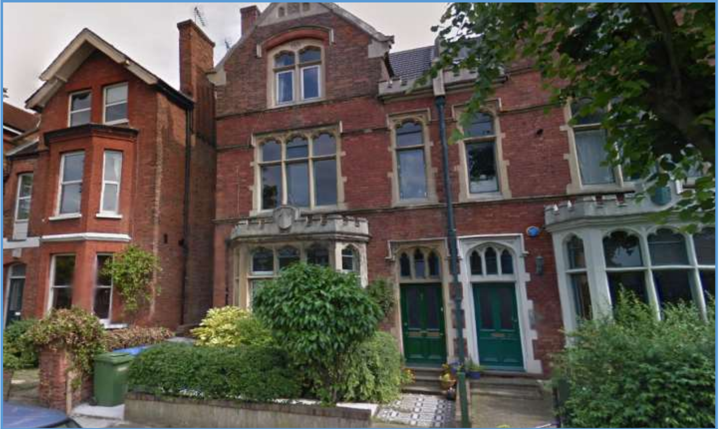
Possible boundary extension to the Willesden Green Conservation Area along Dean Road
