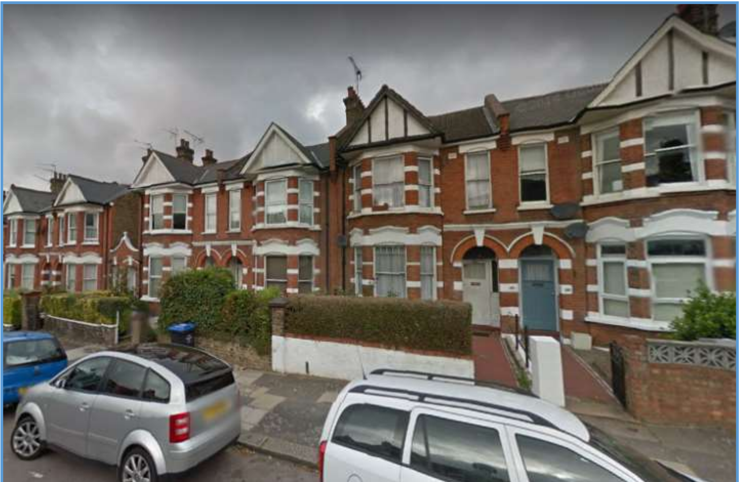
Ridley Road. Decorative Victorian brick terraces with stone dressings and original front doors
