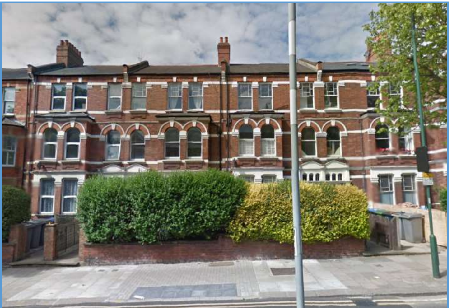
Possible boundary extension along Salusbury Road
