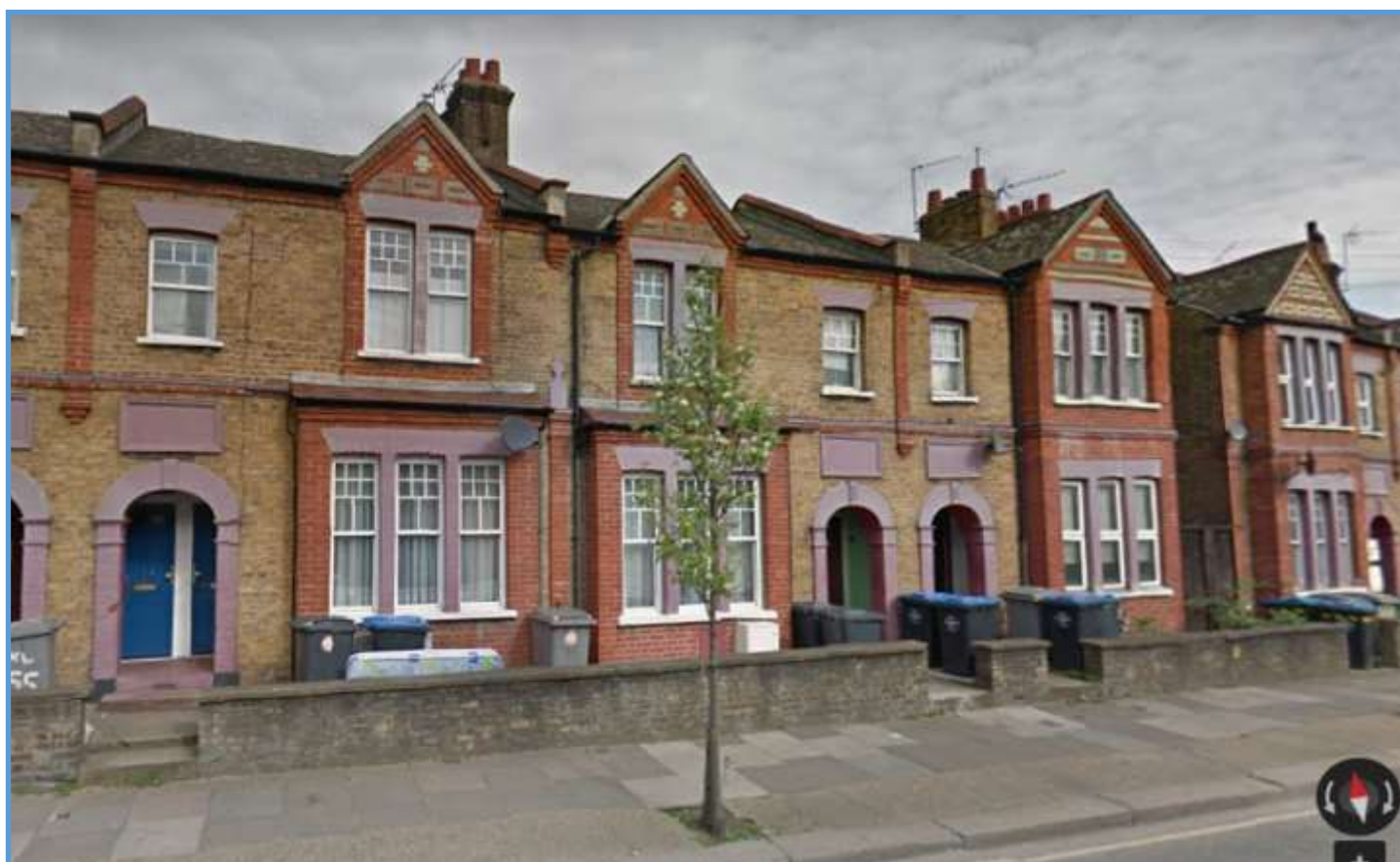
Victorian brick railway cottages constructed for the London and North Western Railway
