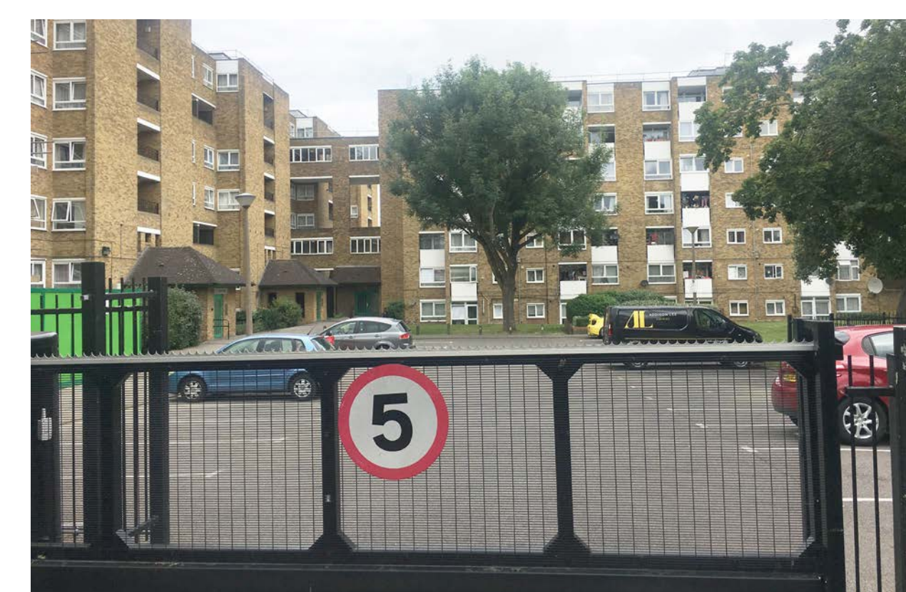
Existing Estate - current railing system
