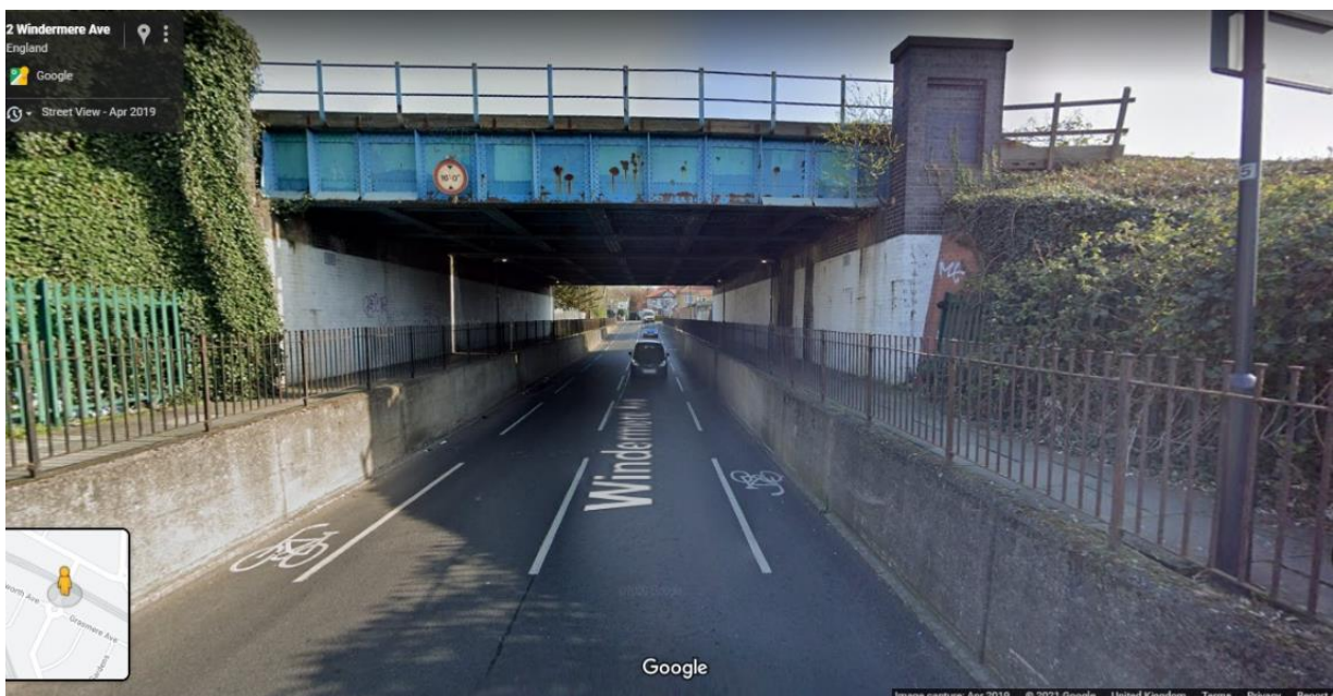
Figure 8 - Windermere Avenue underpass
