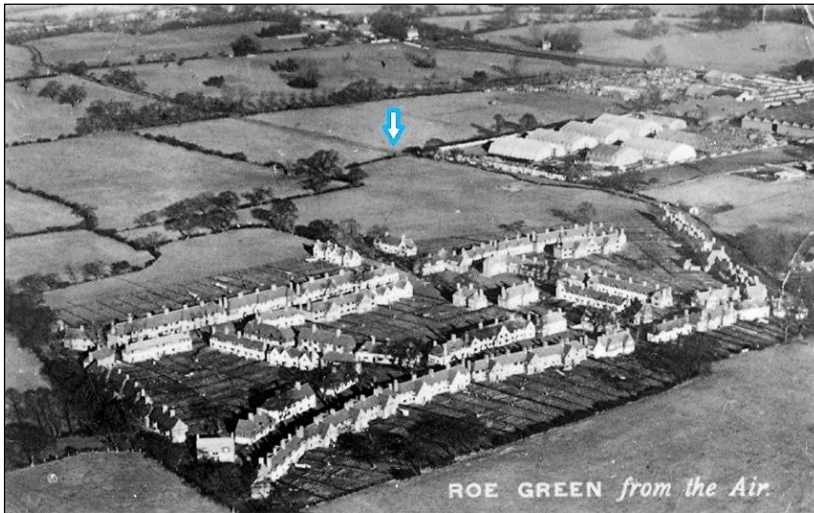
An aerial view of Roe Green Village, c.1920, with arrow showing Stag Lane.
