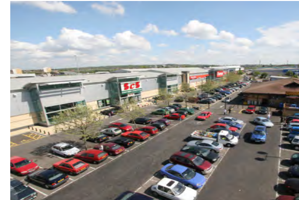
Staples Corner retail park
