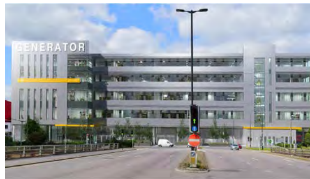
The Generator building, Grand Union Masterplan
