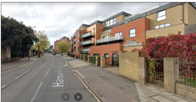
Figure 6: Eastern section looking west towards Kensal Green station; Rhapsody Court on the right.
