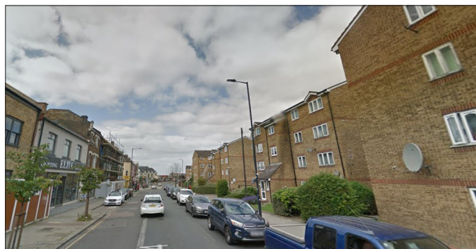
Figure 9: Western section looking west towards Scrubs Lane; Brunel Court to the right; LB Hammersmith & Fulham to the left.
