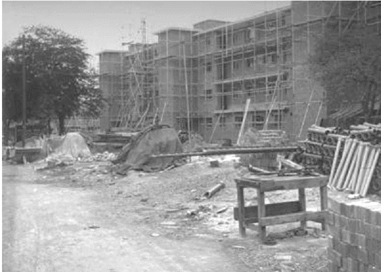
20a. Keneric Court flats under construction, June 1950. [Brent Archives online image 3850]
