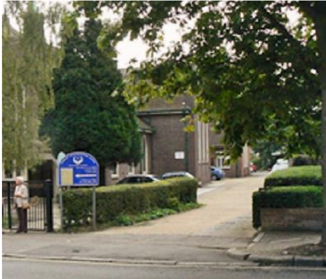
22b. Sudbury Methodist Church, 2015. [Photo by Rod Lake]
