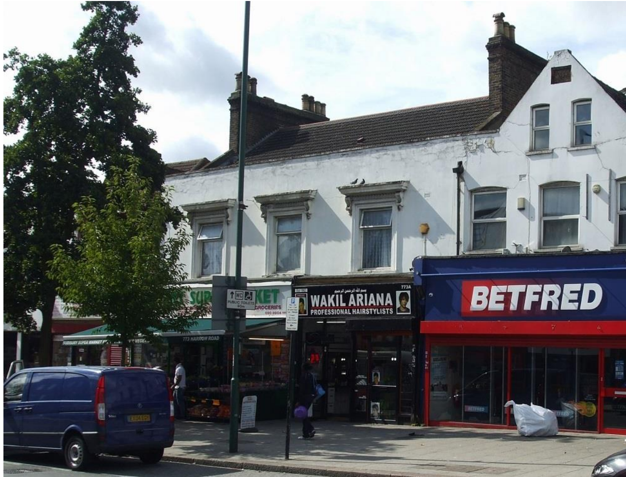
27b. Sudbury Supermarket, Harrow Road, 2015. [Photo by Philip Grant]
