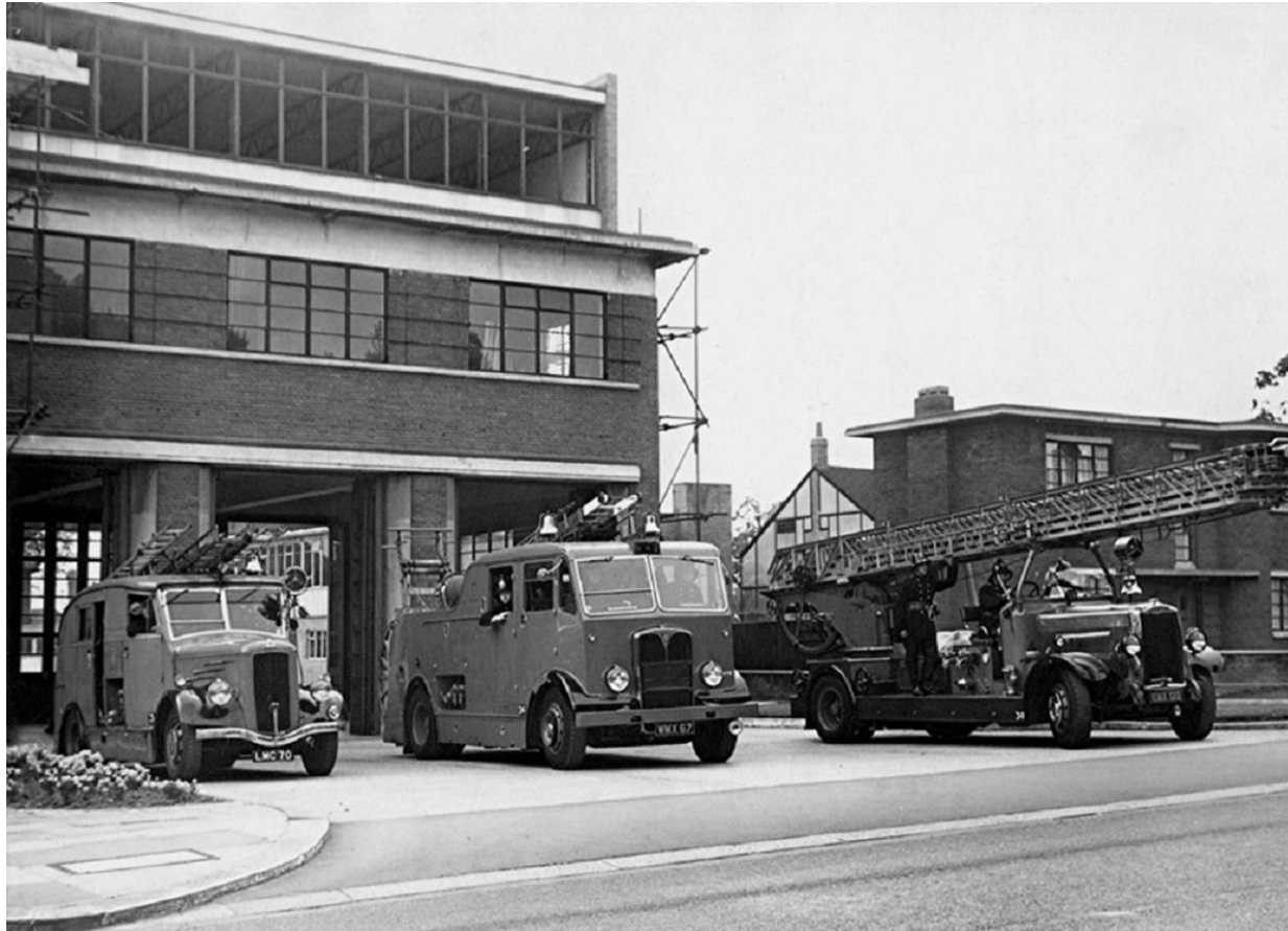
35a. Wembley Fire Station, Harrow Road, 1952. [Photo from Brent Archives]
