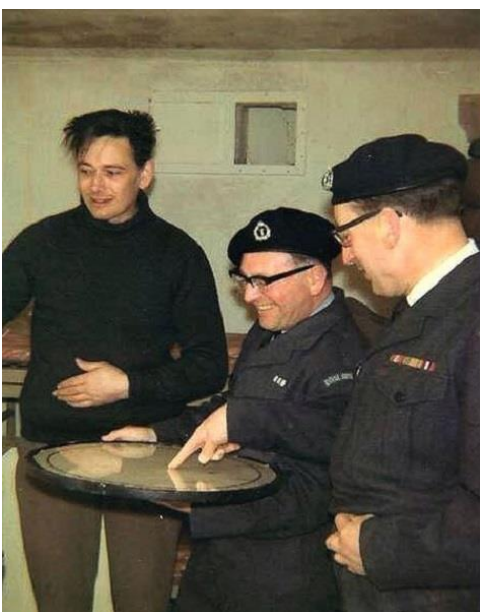
6. Inside the monitoring room in the Gotfords Hill bunker.
