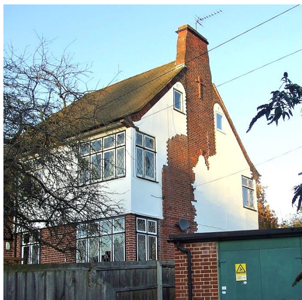
8 Old St Andrew's Mansions, showing its side wall.
