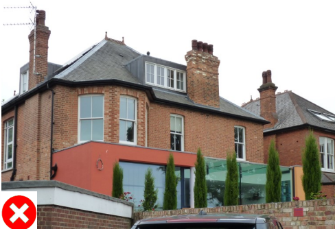
Rear extensions in uncharacteristic materials
