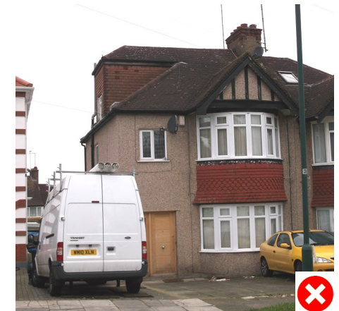
Side dormer that distorts the character of the roof and the building
