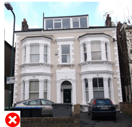
Too large, uncharacteristic front dormer
