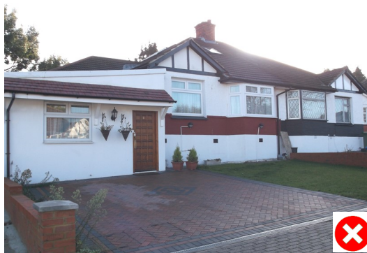
Too wide, protruding, uncharacteristic extension
