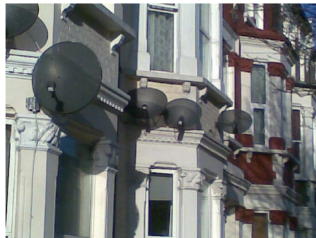
Apartment buildings should provide communal communications facilities ❌
