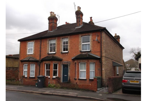
A hipped roof with chimneys ✓
