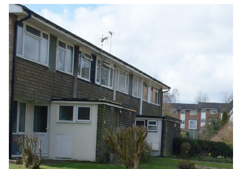
Inactive protruding elements to the front of the building, blocking views from and to ground floor doors and windows ❌
