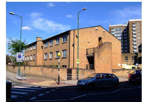
Blank side gables are inappropriate ✗
