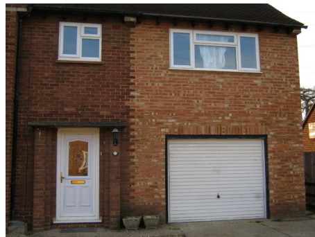
Integral garages cause a lack of active frontage on the ground floor ❌
