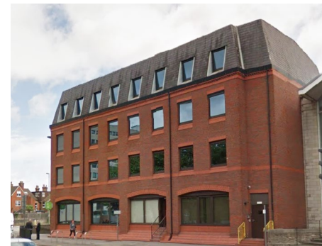
A mansard roof with setback windows ✓
