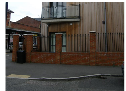
Needlessly high walls and railings reduce the interaction between building and street and give the impression the area is unsafe
