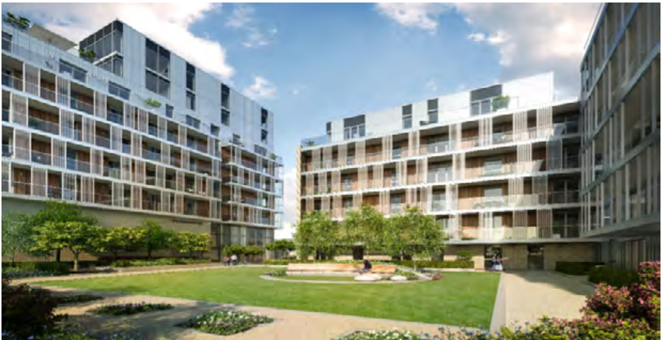
Illustration 2. Queens Park Place - Communal Courtyard
