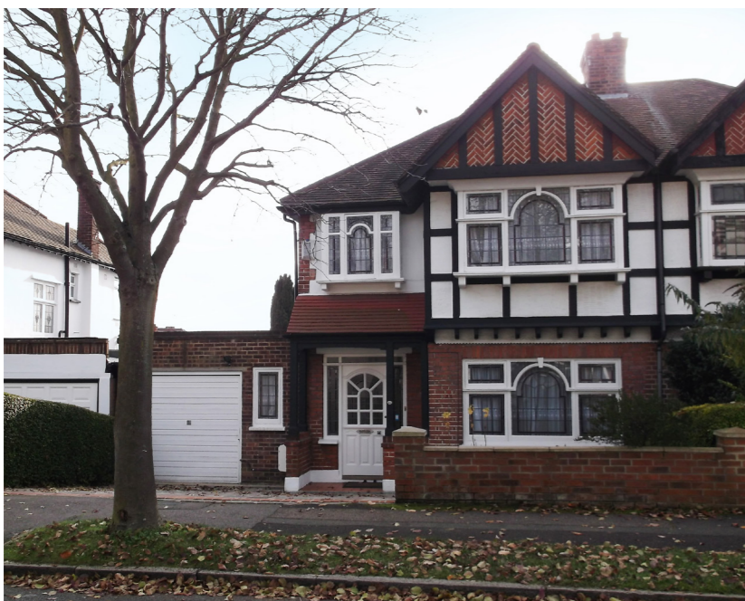
Figure 22: Decorative features at Sudbury Court
