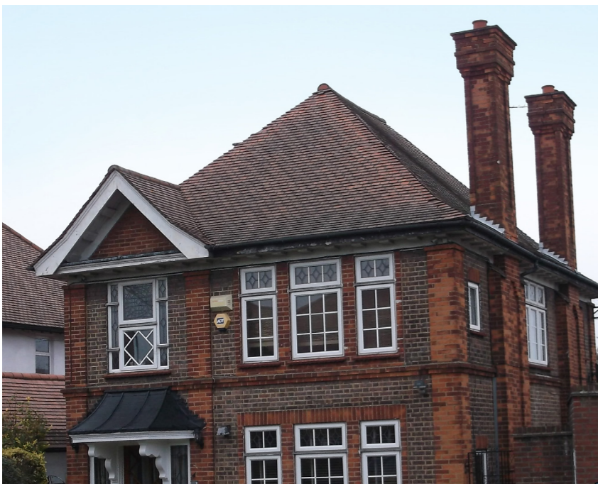
Figure 26: Decorative brick chimney at Sudbury Court
