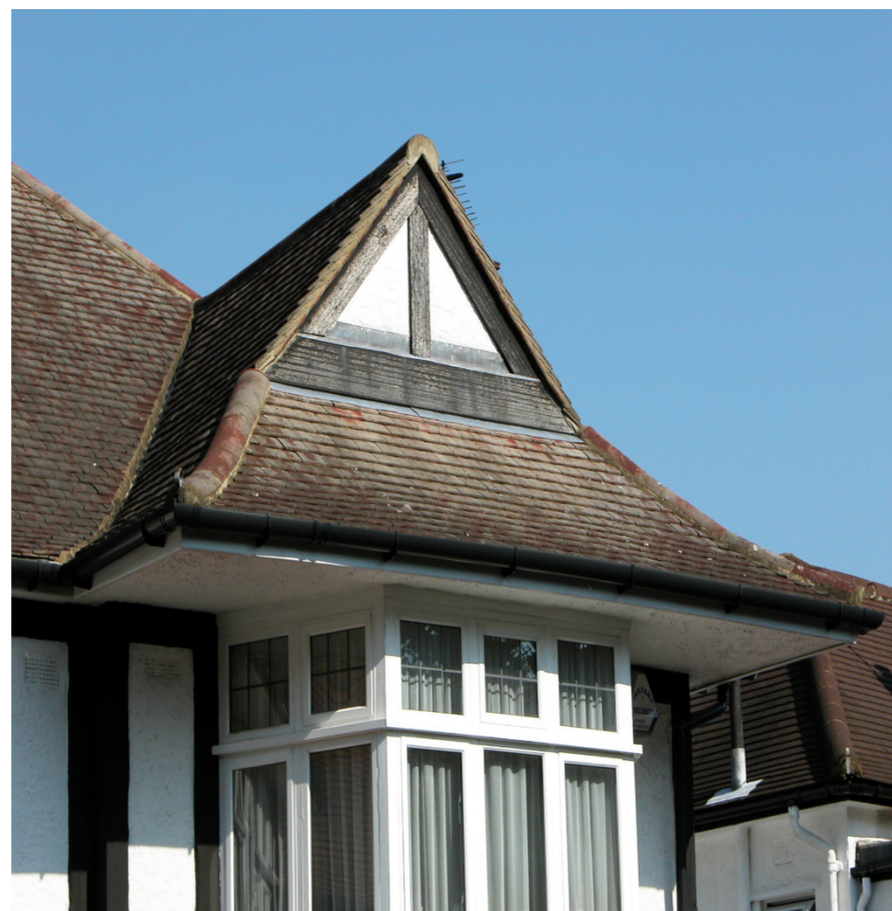
Figure 19: Window details at Sudbury Court
