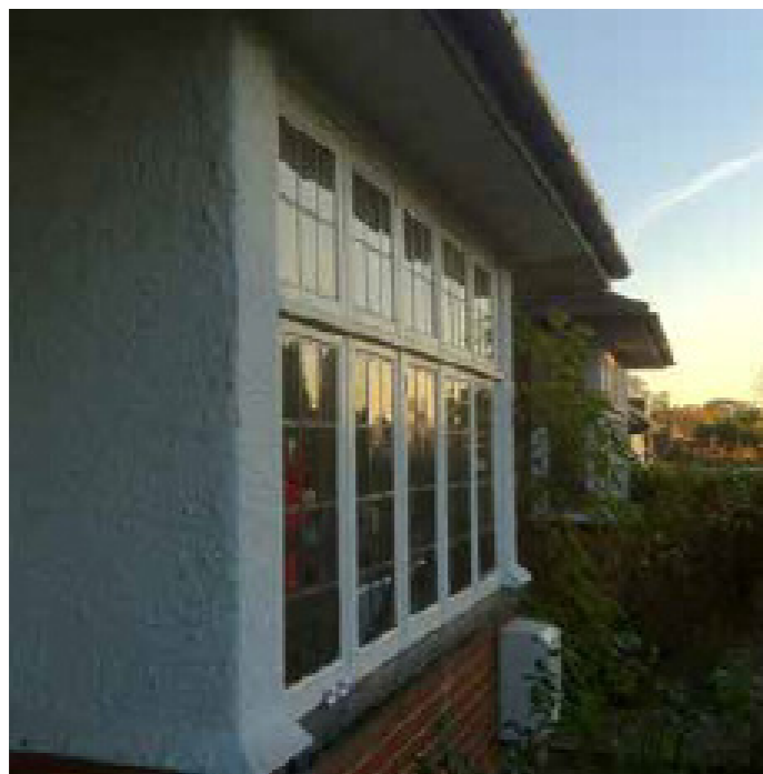
Figure 17: Window details at Sudbury Court
