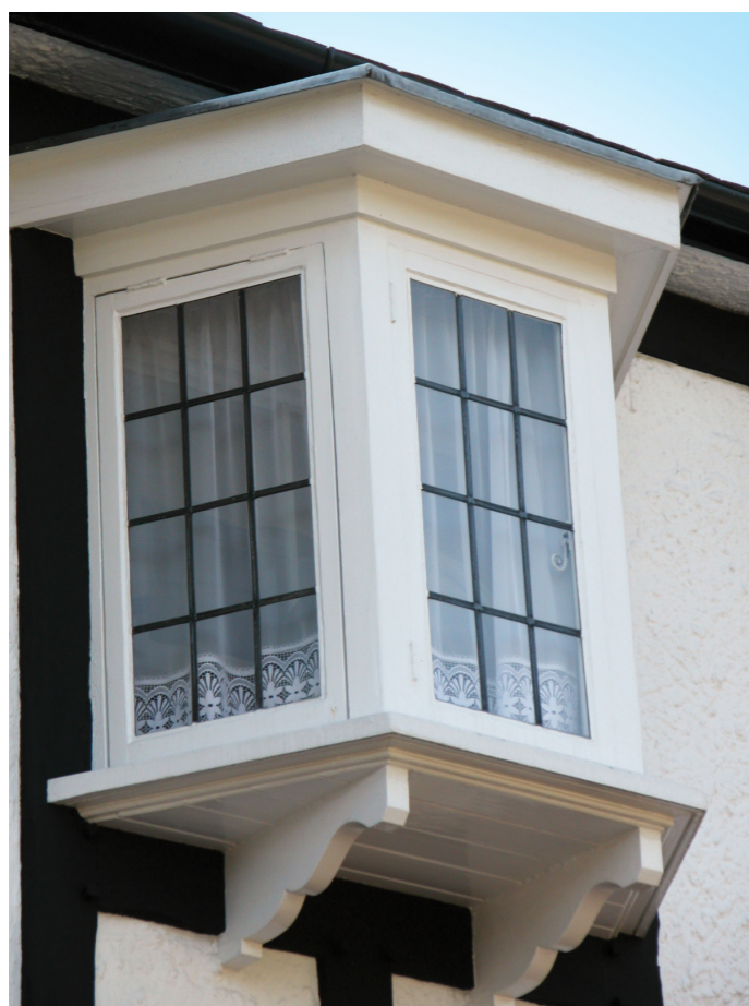
Figure 18: Window details at Sudbury Court
