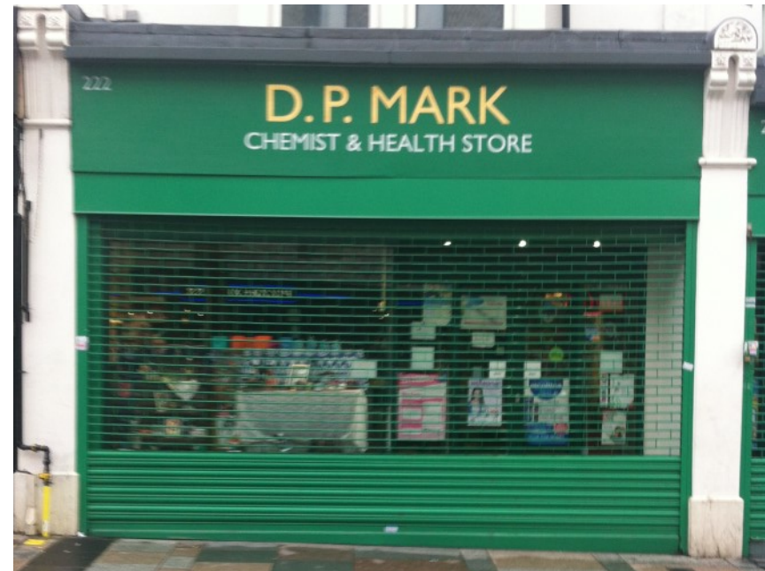
An external shutter of this style will only be acceptable where it can be demonstrated it is necessary for insurance purposes.
