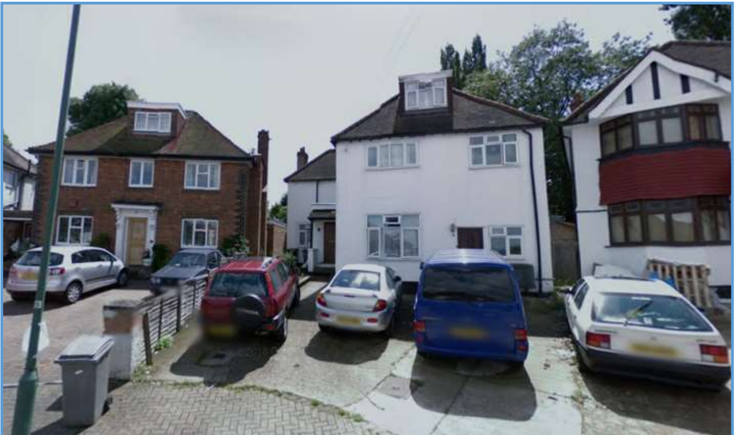
Possible removal of properties from the Buck Lane Conservation Area in Pear Close.
