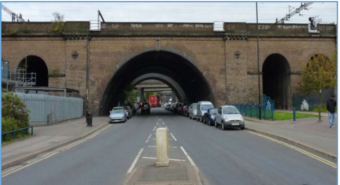
Grade II listed railway bridge, 1838, by Robert Stephenson. Viaduct from the London & Birmingham Railway, carrying the main line from Euston. In the OPDC planning area of responsibility.
