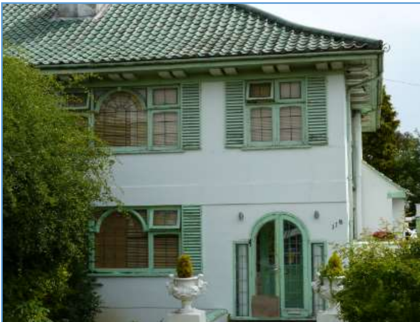
Moderne houses enlivened by bright green pan tiles in the Sudbury Court Conservation Area.
