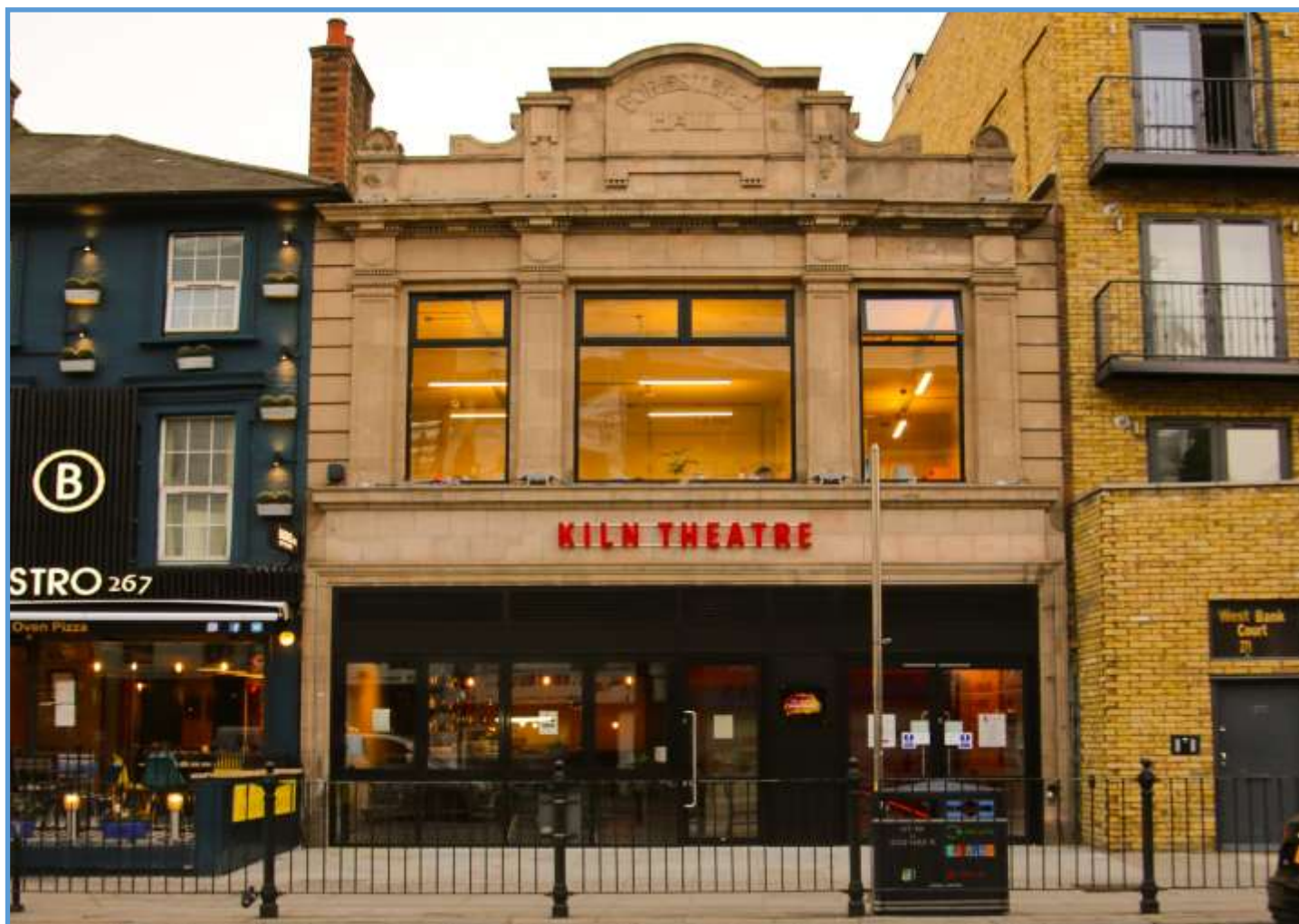
Locally listed Kiln Theatre on Kilburn High Road showing detail of the refurbished 1929 Foresters' Hall façade and new shopfront.
