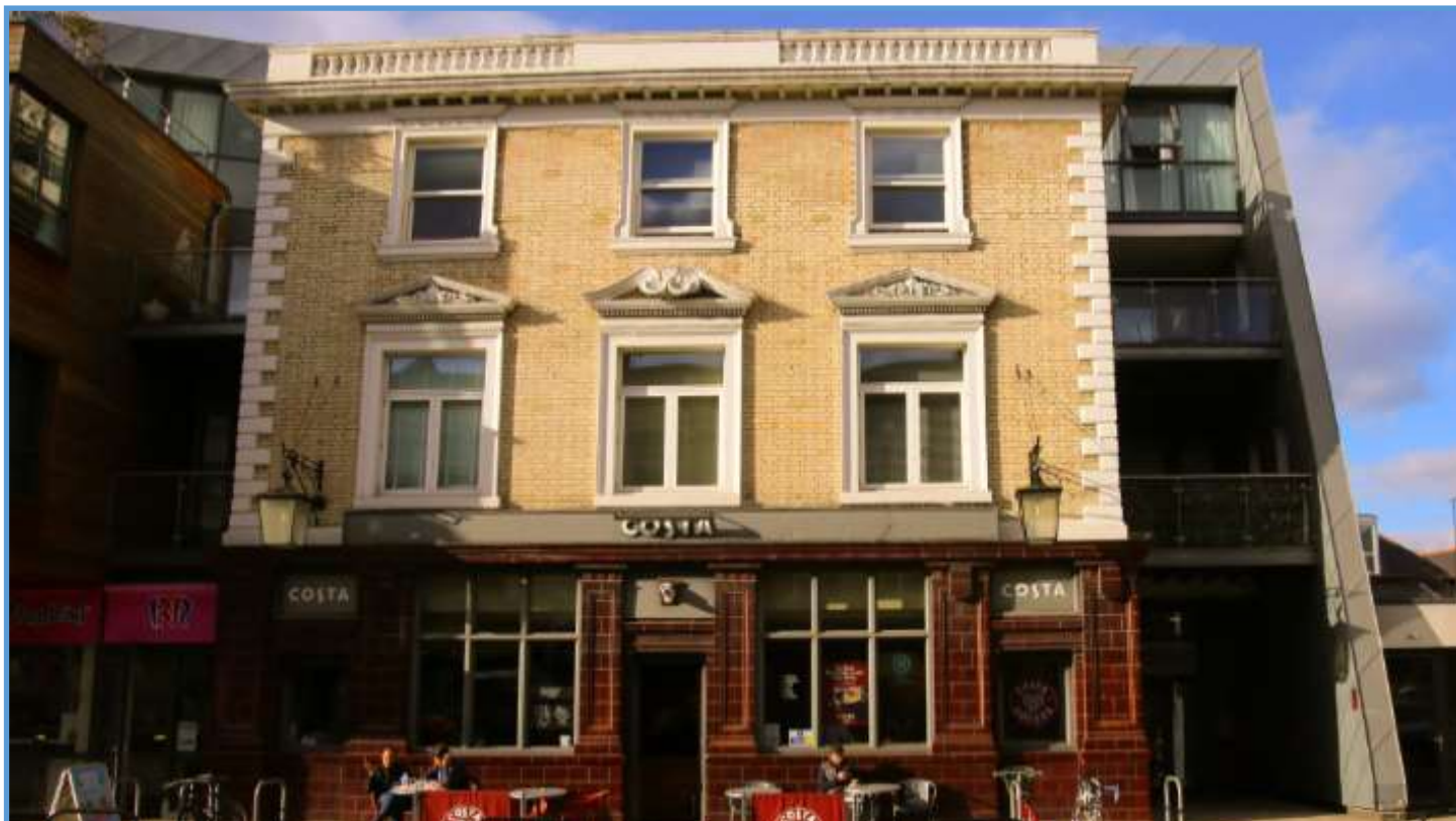
Locally listed former Spotted Dog Pub, High Road Willesden, 1881 by H W Hexton converted and extended for new uses in 2014.
