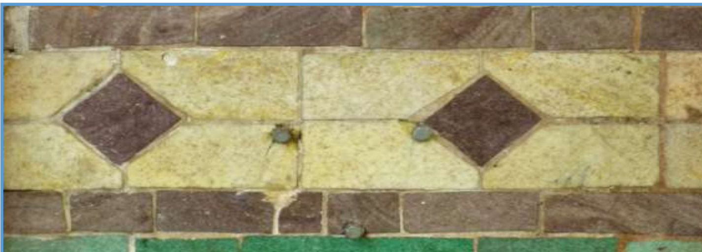
Detail of the glazed bricks within the ticket office at the Grade II listed Willesden Underground station. 1925 by Charles Walter Clark, architect for Metropolitan Railway Company.
