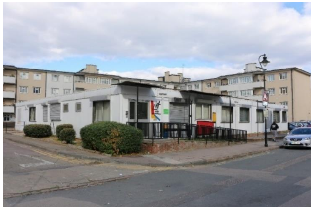
South Kilburn Studios currently provides spaces for SMEs and community ventures. The site is subject to ongoing LRF-funded proposals and tenants are due to be moved to new premises before the end of 2016.
