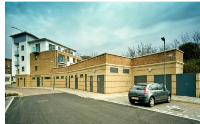
Harrow Road ACME artist studios were delivered in 2010 in partnership with the Kensington Housing Trust who manage the affordable residential units on the upper level.
