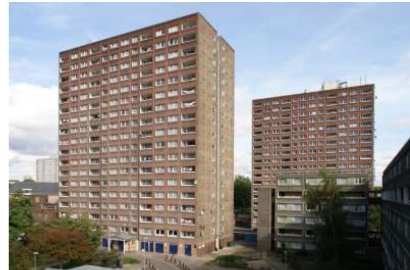
Two of the tall buildings scheduled for demolition
