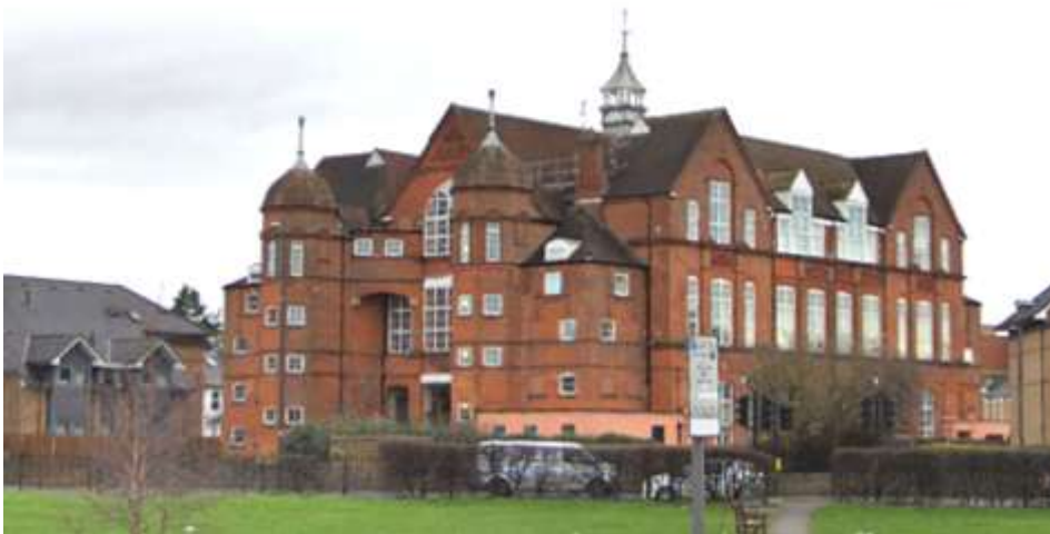
Locally listed Shortcroft Mead Court on Dudden Hill Lane, adjacent to the site
