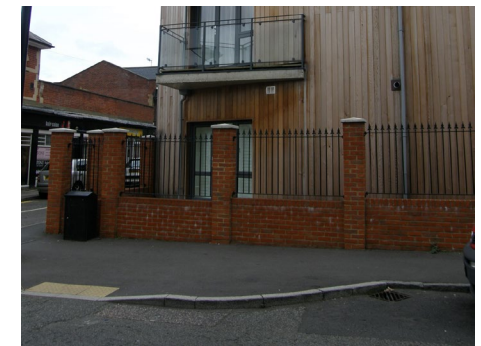
Needlessly high walls and railings reduce the interaction between building and street and give the impression the area is unsafe
