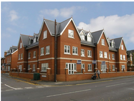
A varied roofscape and depth that breaks the building into smaller parts ✓
