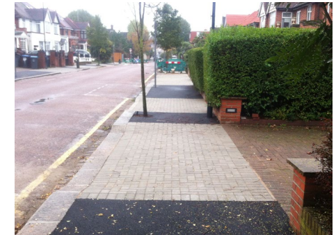
Concrete block paving creating a durable and attractive footpath surface ✓
