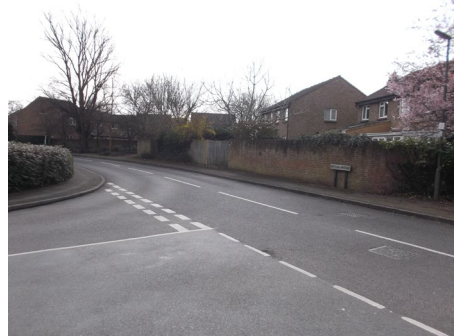
A collector road should still have building frontage, cycle lanes and pedestrian crossing facilities ✗
