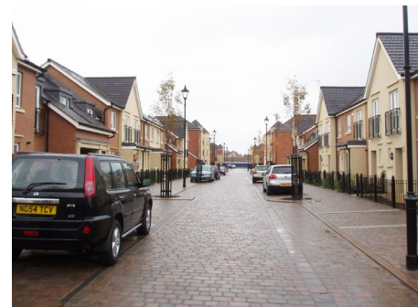
Local street with attractive materials, planting and on-street parking ✓
