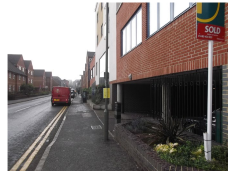
Undercroft parking in inappropriate location creating inactive frontage ✗
