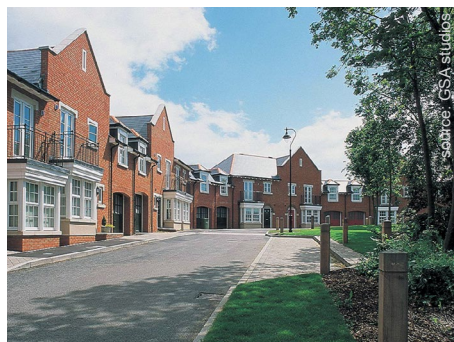
Animated facades with bay windows ✓
