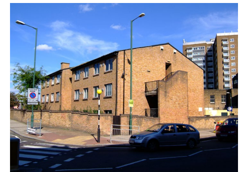
Blank side gables are inappropriate ✗
