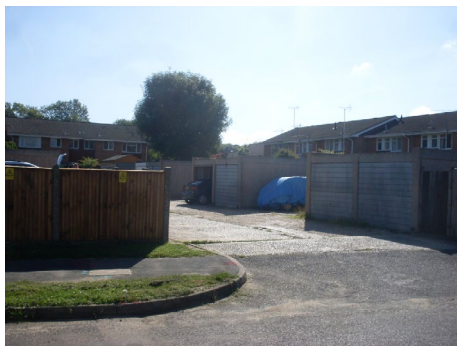
Rear parking street causing inactive space without supervision of cars or people ❌
