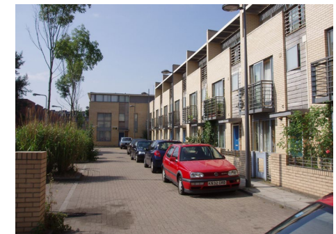
Local street with attractive materials, planting and on-street parking ✓
