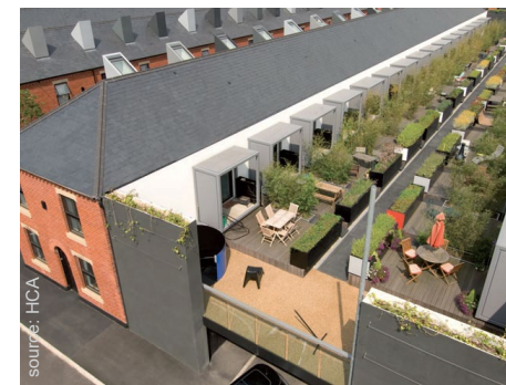
An innovative example of under-deck parking, providing garden space above parking for a traditional terrace ✓
