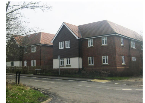
A lack of ground floor entrances and private front gardens creates an inactive street ✗
