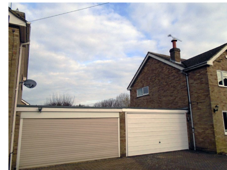
Double garages are rarely used for parking and cause inactive frontage ❌
