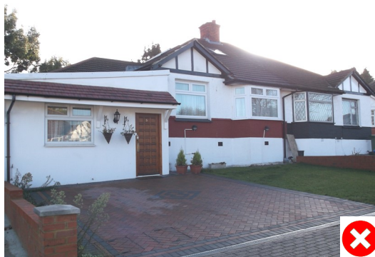
Too wide, protruding, uncharacteristic extension
