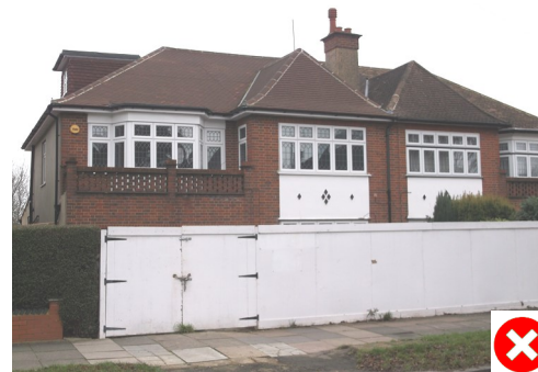
High fence along the street, creating inactive frontage
