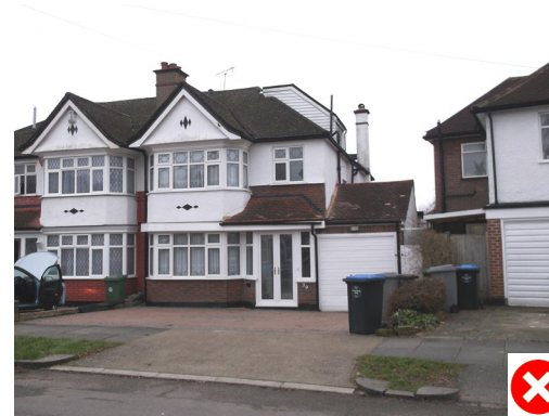
Fully paved front garden, using tarmac
