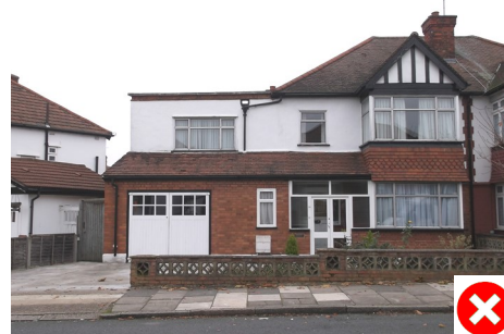
Protruding ground floor and first floor not set back from the main wall
