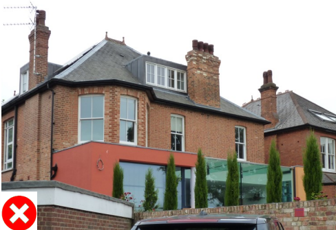
Rear extensions in uncharacteristic materials
