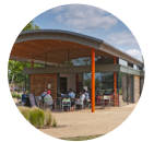
Park building and hard-space
