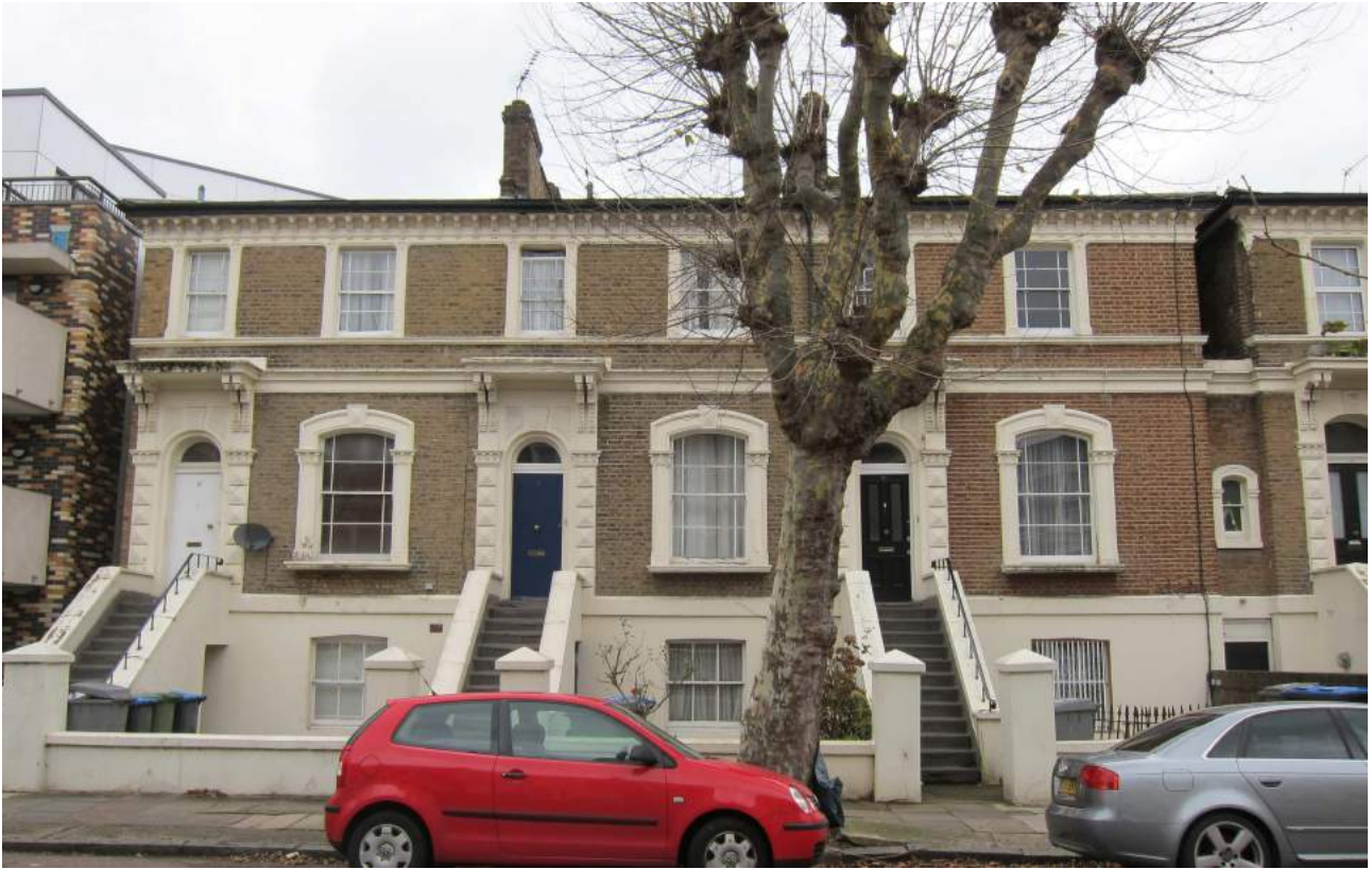
Street elevations – 9 Princess Road on right, 13 Princess Road on right
