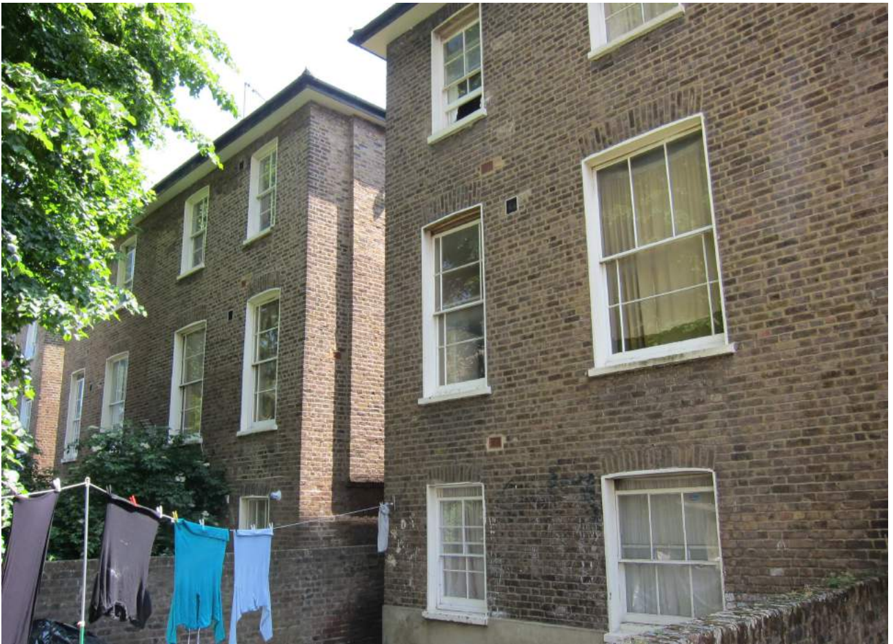
Rear elevations -17 Princess Road on right, 19 - 23 Princess Road beyond
