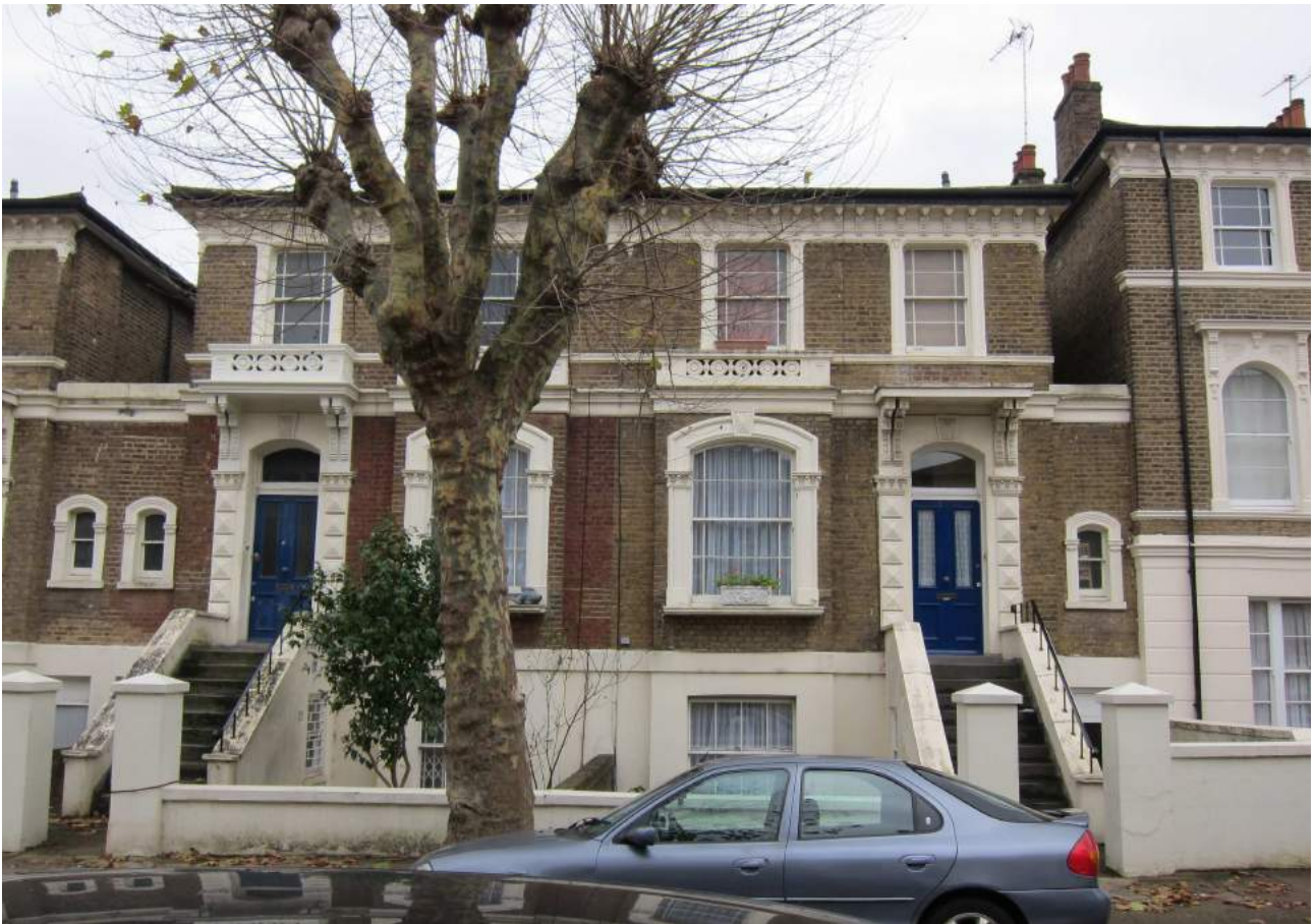
32 Princess road on right, 34 Princess Road on left
