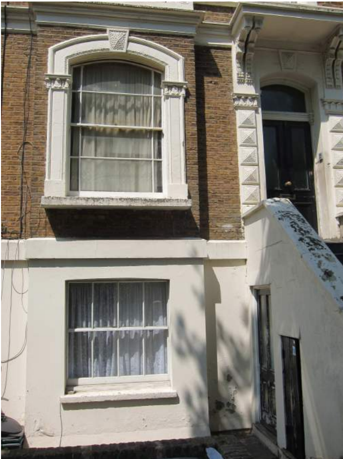
Typical street elevation ground and first floor windows
