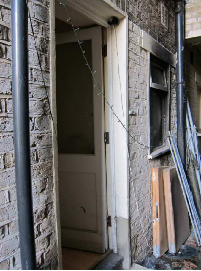
Ground floor side elevation garden door (15 Princess Road)
