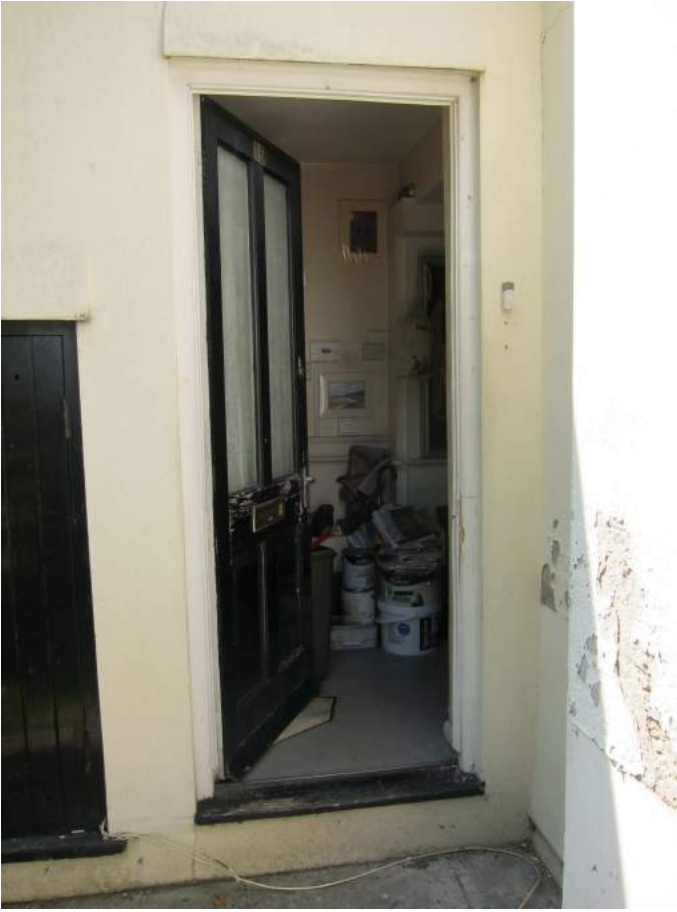
Typical ground floor flat entrance door (15 Princess Road)
