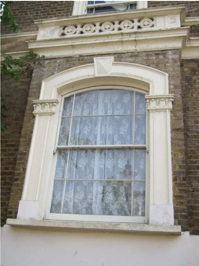
Street elevation first floor window to 84 Princess Road
