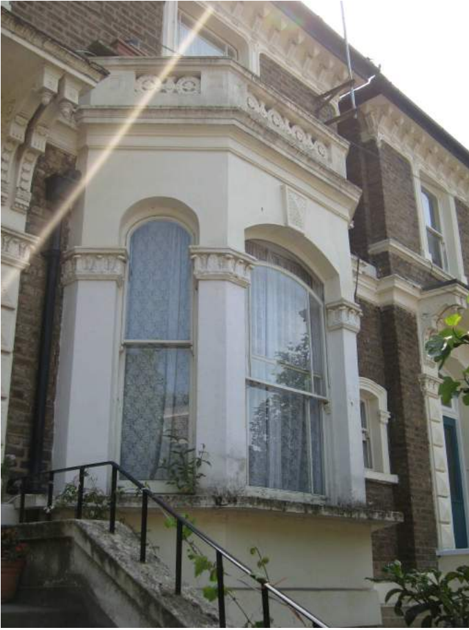
Street elevation first floor bay window to 84 Princess Road
