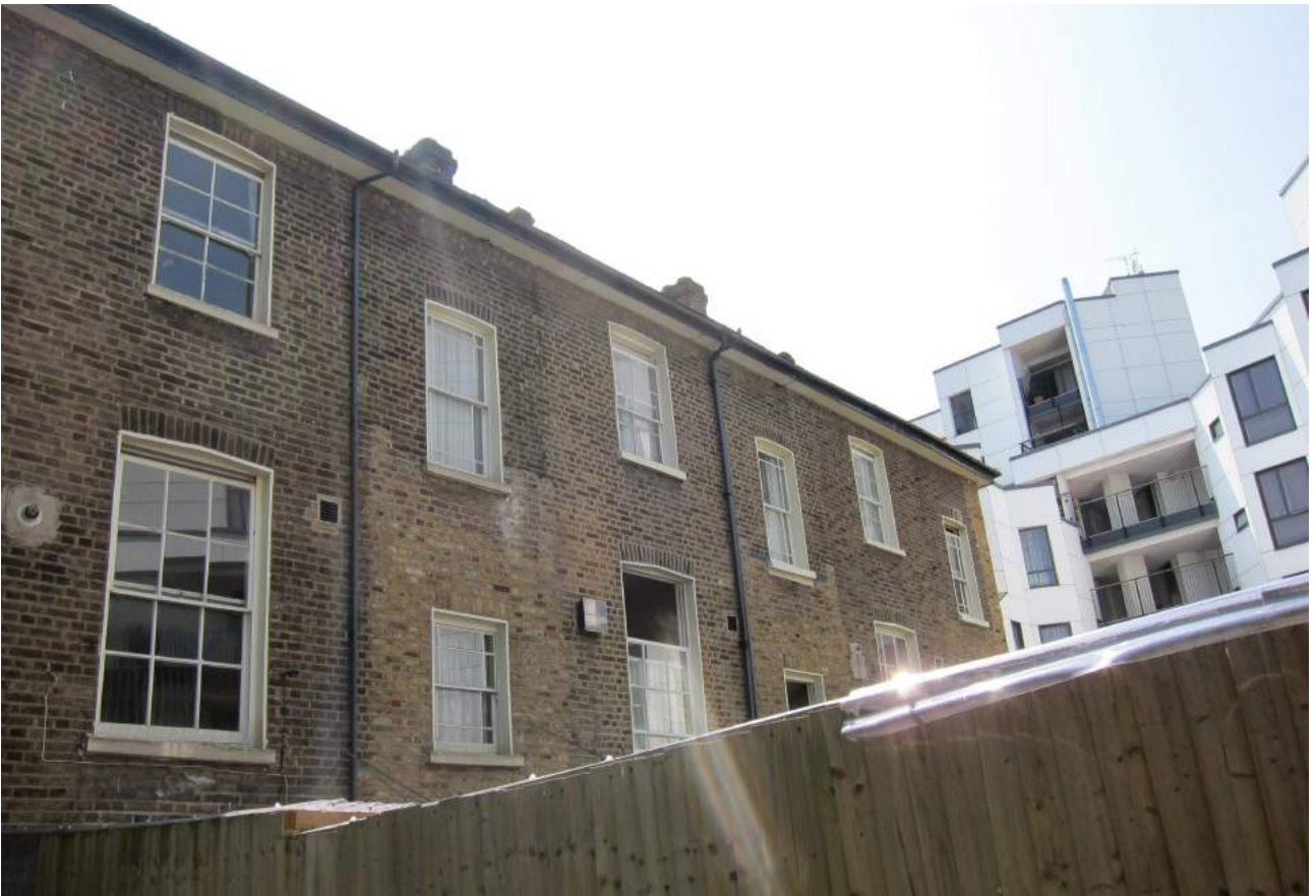
Rear elevations -13 Princess Road in foreground, 9 Princess Road on right
