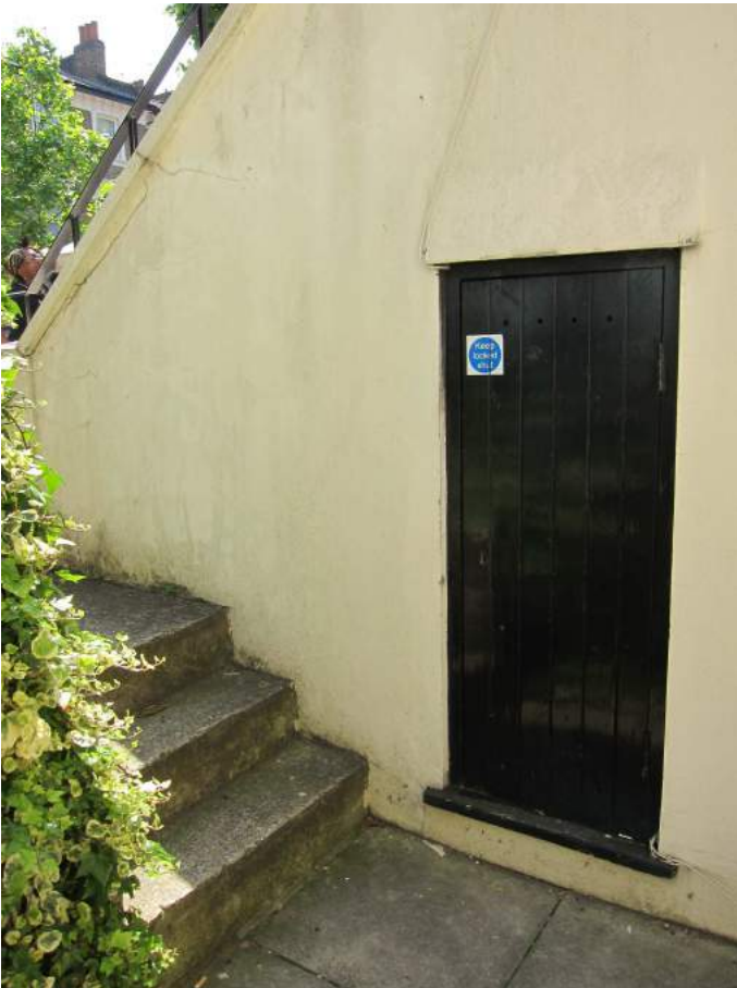
External store/ intake room door below entrance steps
