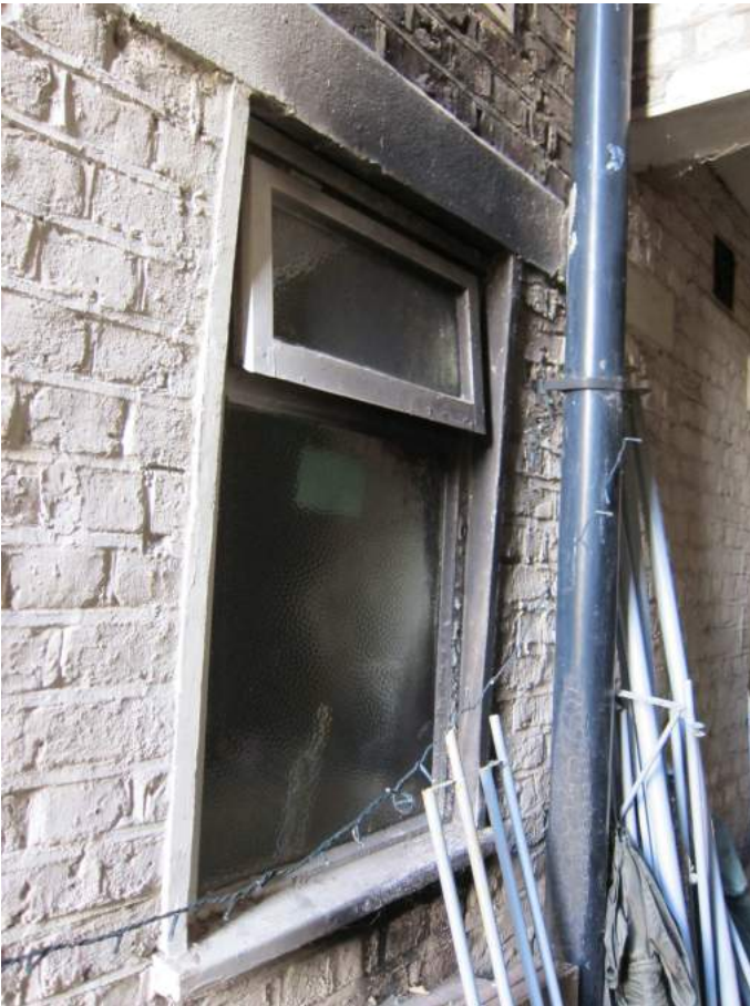
Ground floor side elevation bathroom window (15 Princess Road)
