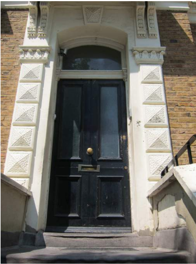
Typical front entrance door at first floor level (17 Princess Road)
