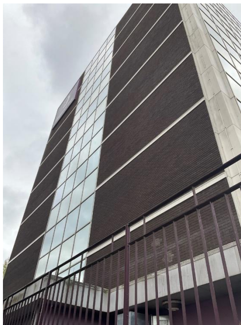
Plate 8: 6-storey hotel building with red and concrete, looking north-east
