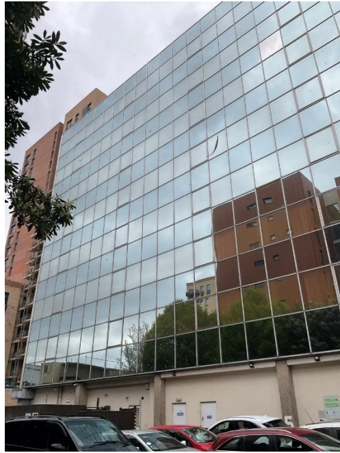
Plate 9: Glass cladding on building, looking north-west
