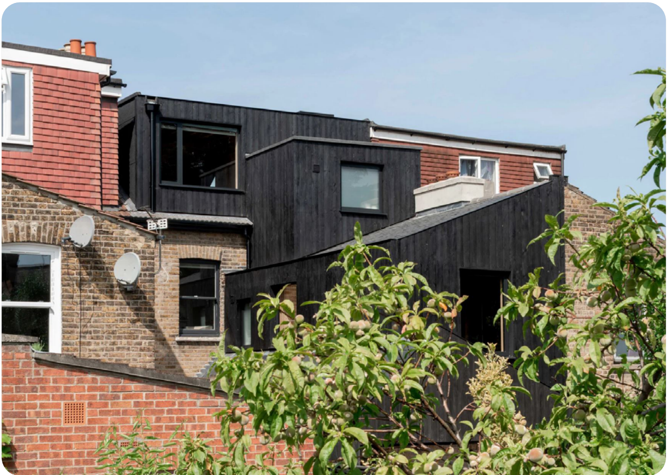
Figure 20: Example of a well designed massing of an L shaped dormer in Walthamstow by Gresford Architects
