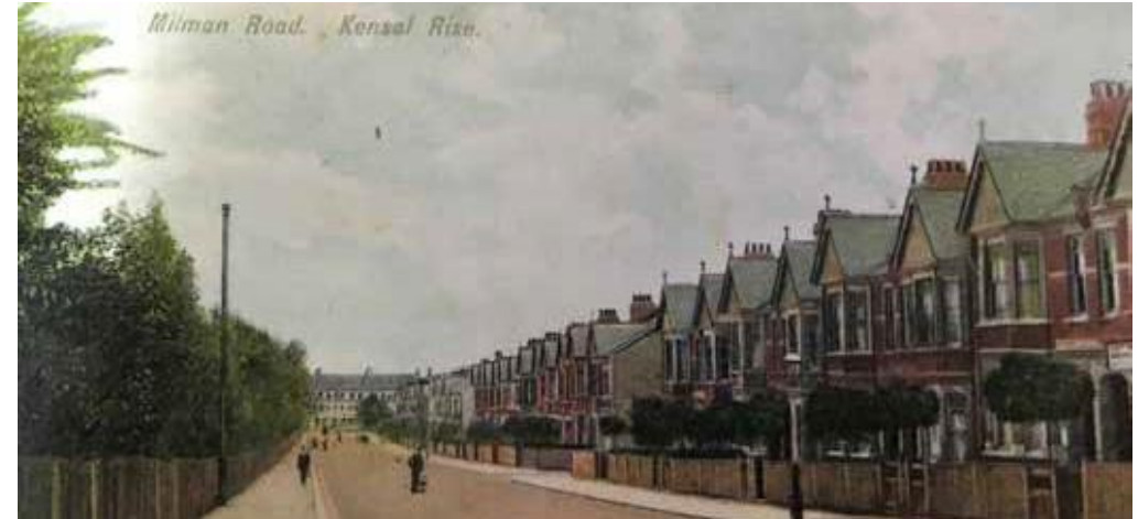
Figure 10: Milman Road in 1907
