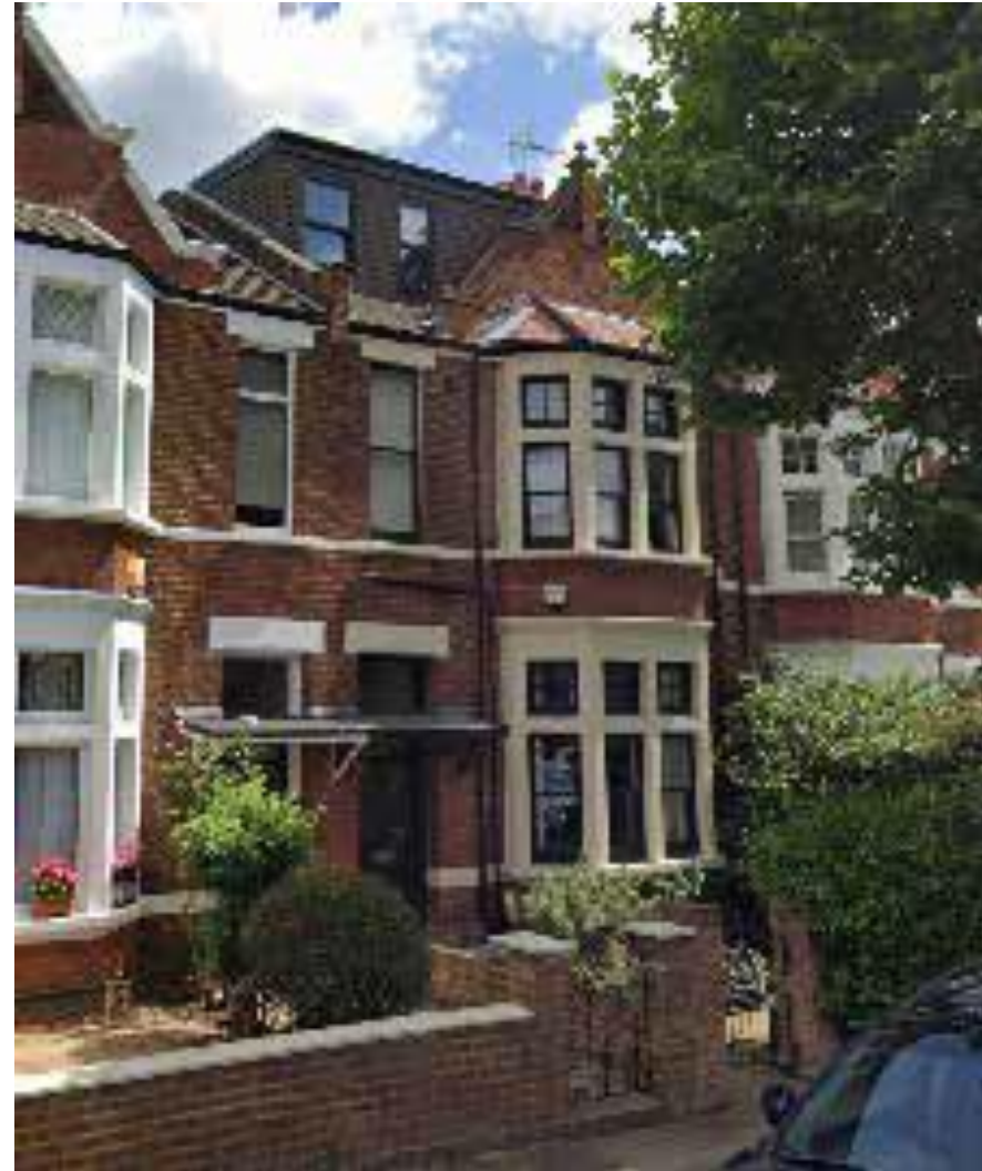
Figure 31: Dormer extension, Dundonald Road
