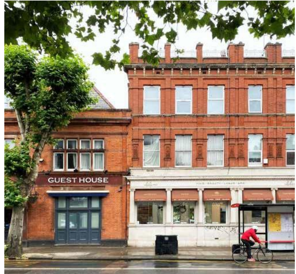
Figure 13: The Windmill hotel building adjacent to 59-61 Cricklewood Broadway that make a positive contribution to the character of the area
