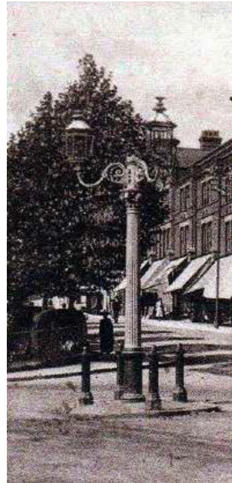
Figure 22: Lampost on Chamberlayne Wood Road c1906
