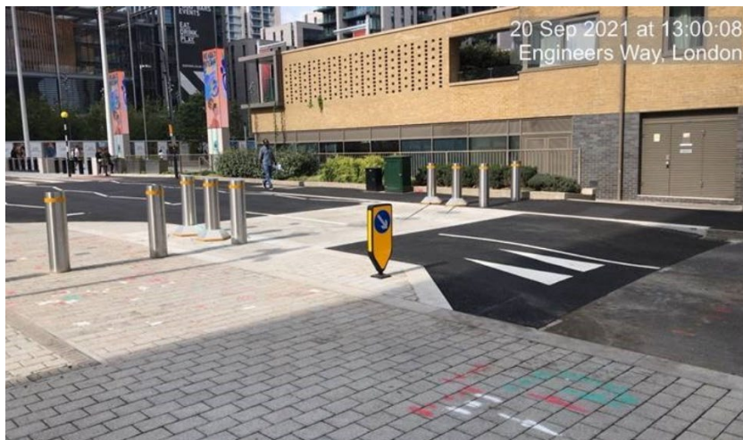
Example of one of the HVM Measures on Engineers Way (Source: LBB)
