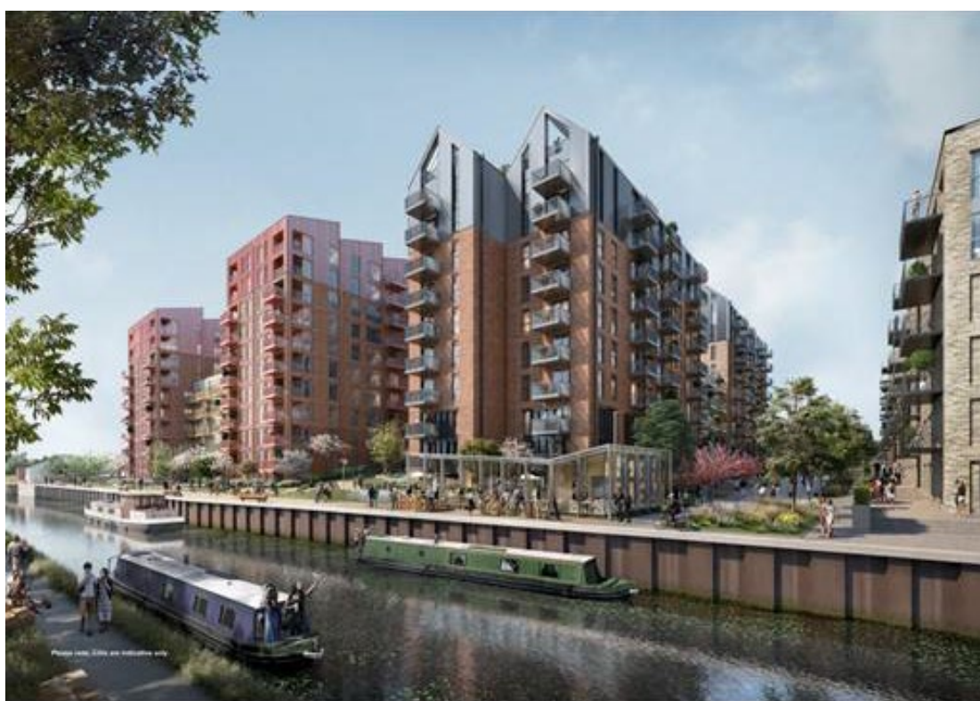
Abbey Manufacturing Estate (Source: Zed Homes Ltd c/o Bell Cornwell LLP, architects Broadway Malyan)
