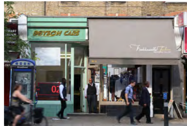
Walworth Road - timber shopfront repair
