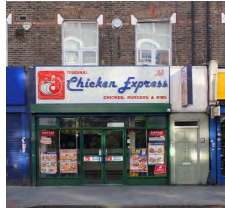
✘ BEFORE: A poorly proportioned 'box' sign, ill-placed projecting sign, visually confusing residential entrance, missing corbel and bracket detract from the shop front's appearance, while large posters on window block views inside the shop
