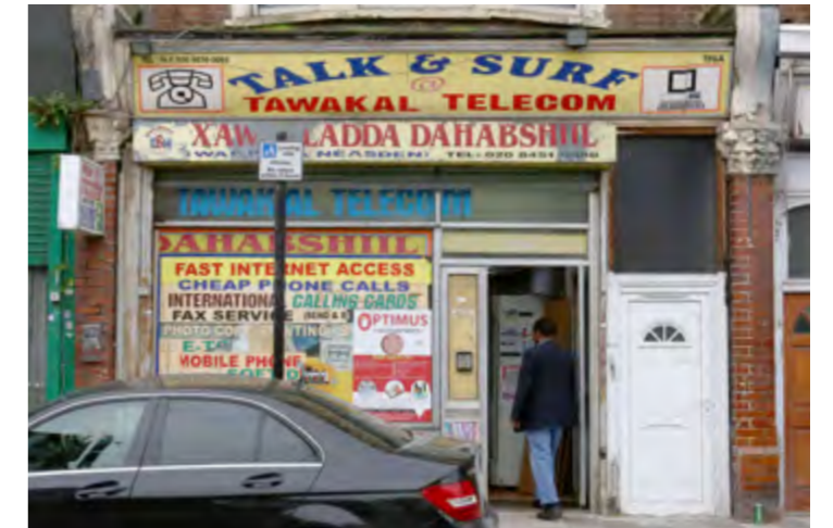
Church Road - cluttered shopfront
